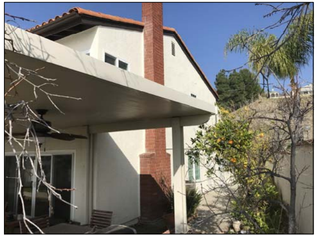
EXISTING HOUSE VIEW B
