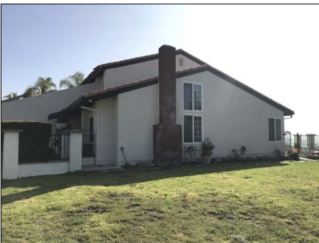
EXISTING HOUSE VIEW D
