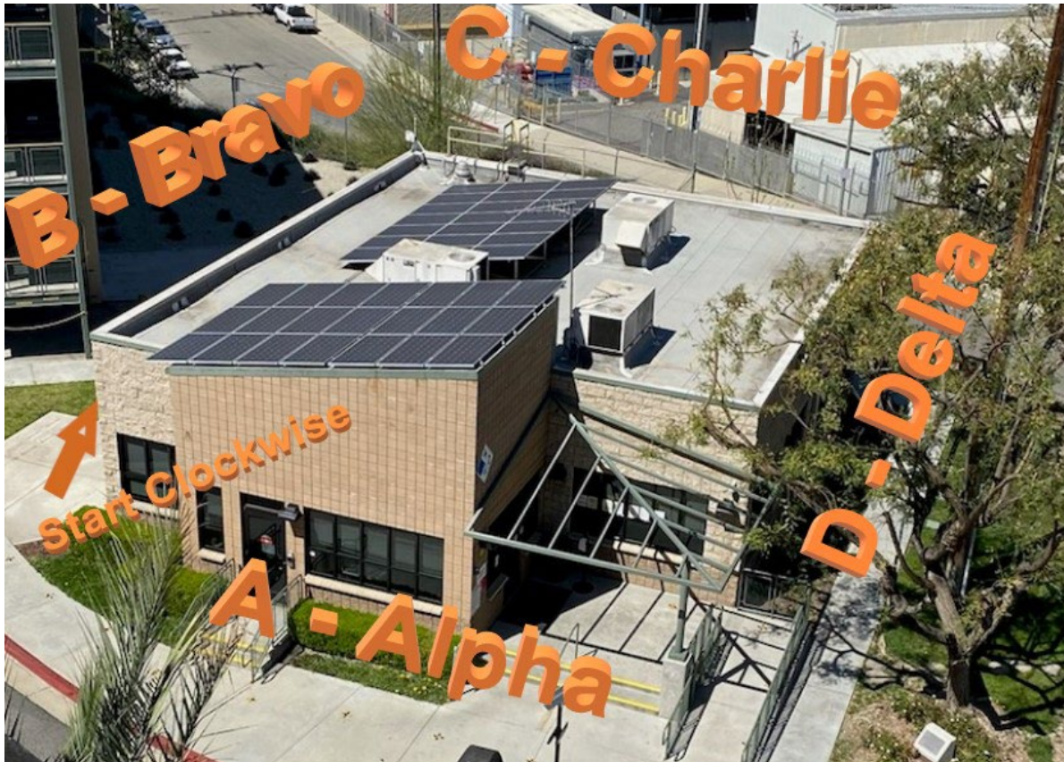
Figure 1. Indexing of a structure (Photo: Captain Donnelly GFD)
