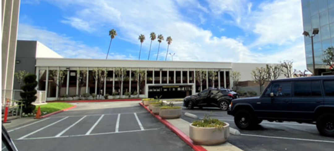
Figure 1: Parking Garage at 620 North Brand Boulevard, view east. Note the simple base, filleted shaft separated by screens and the bracketed, wide upper frieze. The stepped out, framed entry portal on the right-hand side further echoes the Corporate Modern design style of the main building it was constructed to serve. Photograph January 2022.
