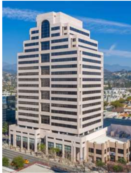
Figure 7: Rendering of 550 N Brand Boulevard, a 21-story building designed by HOK, Inc. and completed in 1989. It is located on the block immediately south of the proposed project. Note the five generous major steps in the design, as well as the different window rhythms, shapes and sizes of openings, the inverted entrance and corners that reduce the perceived mass of the Post-Modernist style building. Not for publication.
