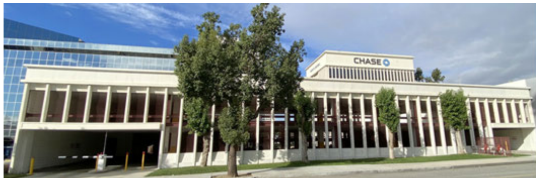
Photograph 2: Home Savings Parking Garage, panoramic view west. The same vertical fins, understated entrance and continuous sign band are that the top. The Building is on right with same sign band. Photograph J. Wilson.
