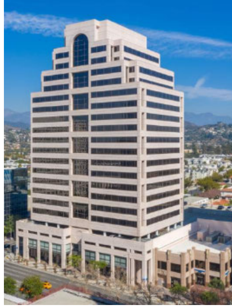
Figure 7: Rendering of 550 N Brand Boulevard, a 21-story building designed by HOK, Inc. and completed in 1989. It is located on the block immediately south of the proposed project. Note the five generous major steps in the design, as well as the different window rhythms, shapes and sizes of openings, the inverted entrance and corners that reduce the perceived mass of the Post-Modernist style building. Not for publication.
