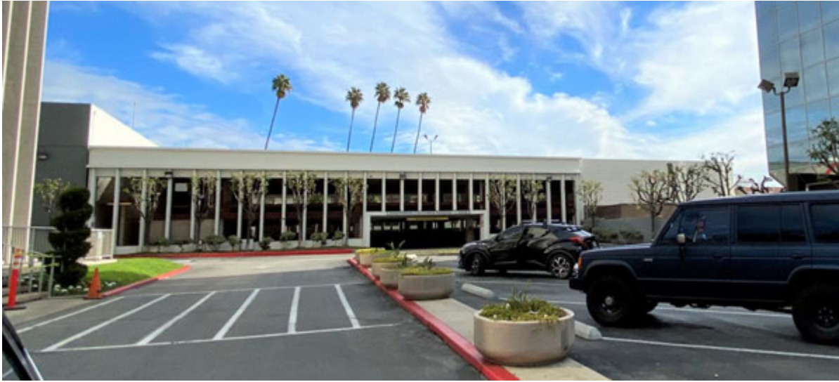
Figure 1: Parking Garage at 620 North Brand Boulevard, view east. Note the simple base, filleted shaft separated by screens and the bracketed, wide upper frieze. The stepped out, framed entry portal on the right-hand side further echoes the Corporate Modern design style of the main building it was constructed to serve. Photograph January 2022.
