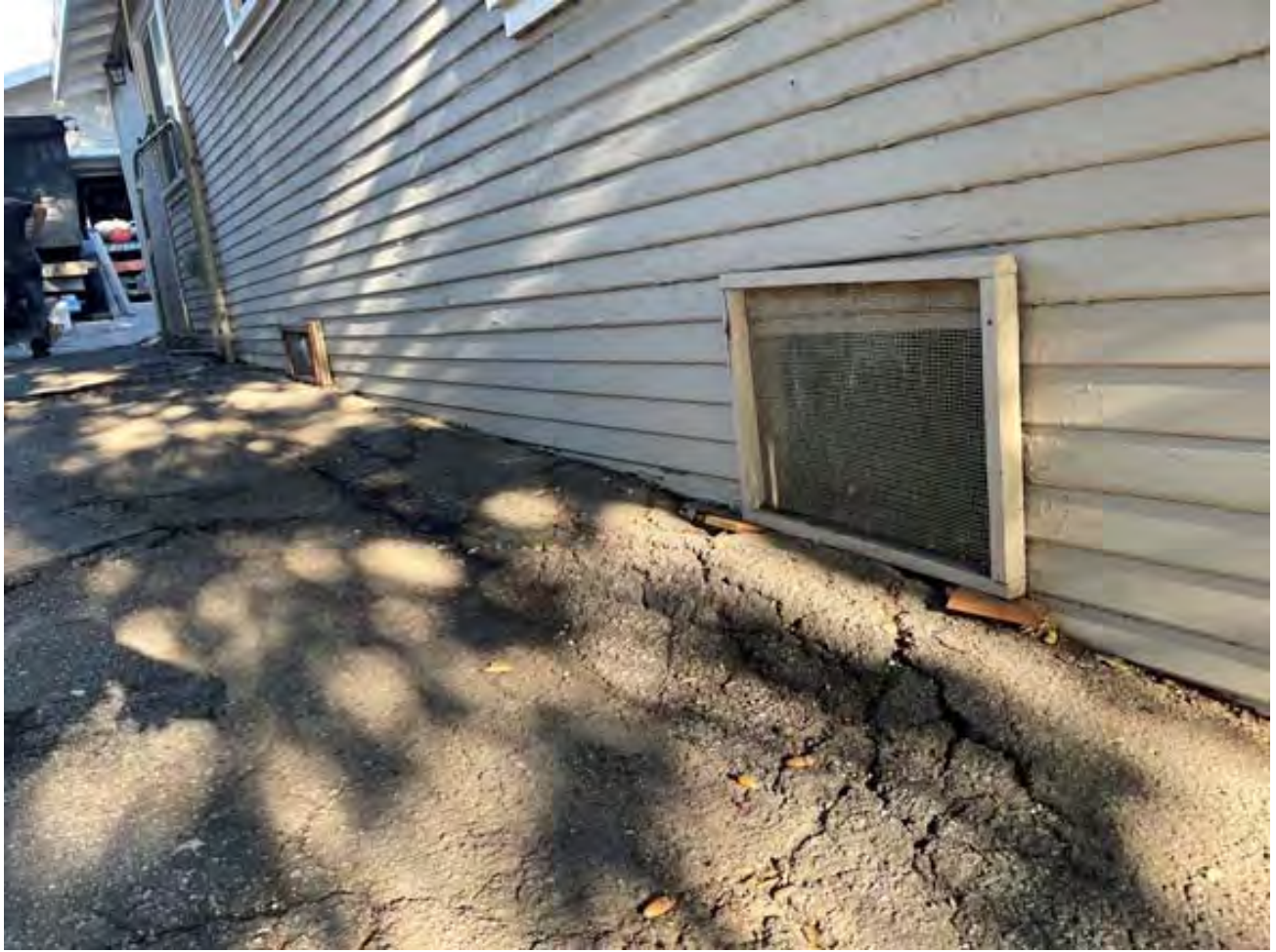
Figure 4: Displacement of the driveway extends from Tree 1 to the side of the existing home. It is likely that some roots grow underneath the home.
