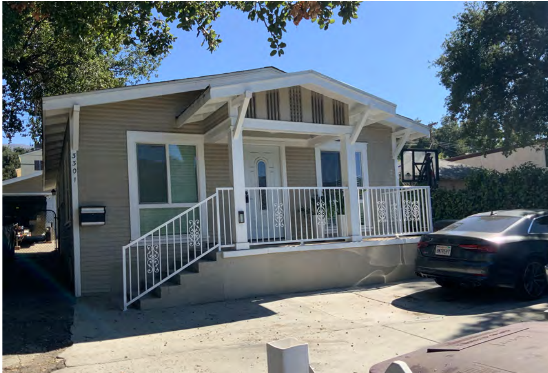
1. SOUTH FACADE LOOKING NORTH FRONT PORCH
