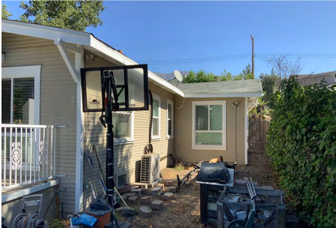
3. EAST FACADE LOOKING WEST
