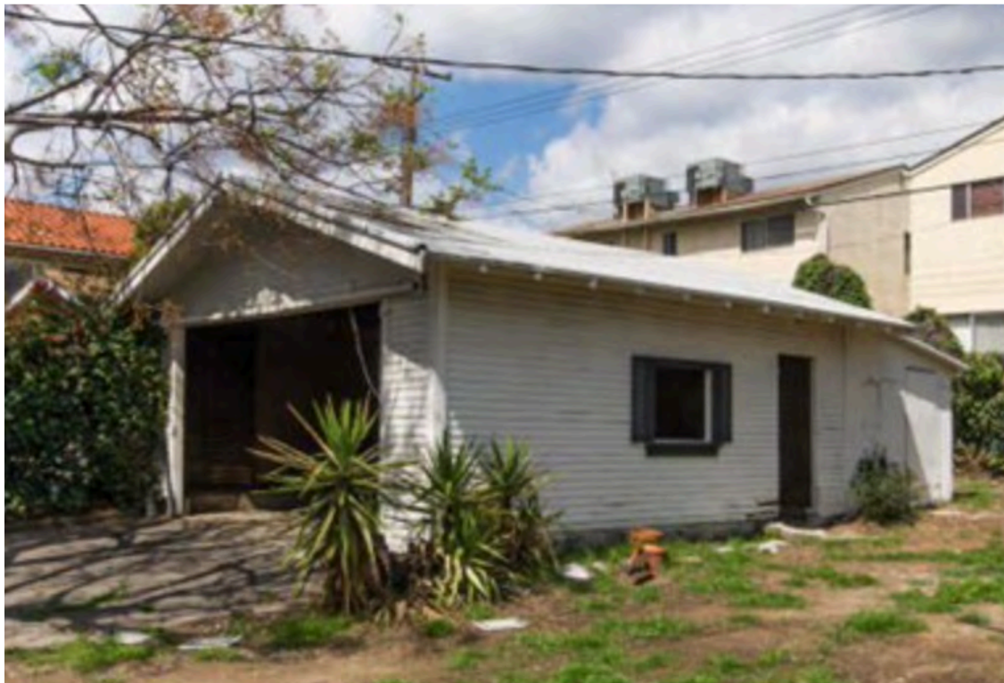
6. SOUTH EAST GARAGE FACADE
