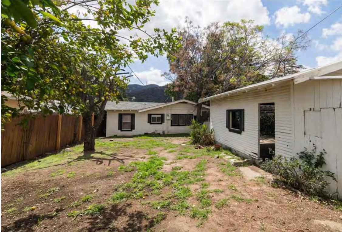
5. EAST GARAGE FACADE
