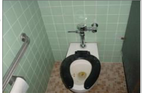
Men's Restroom Across from the Little League Field
