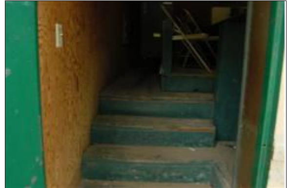
Interior Stairs to the Press Box
