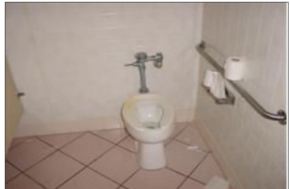
Women's Restroom at the Dad's Club
