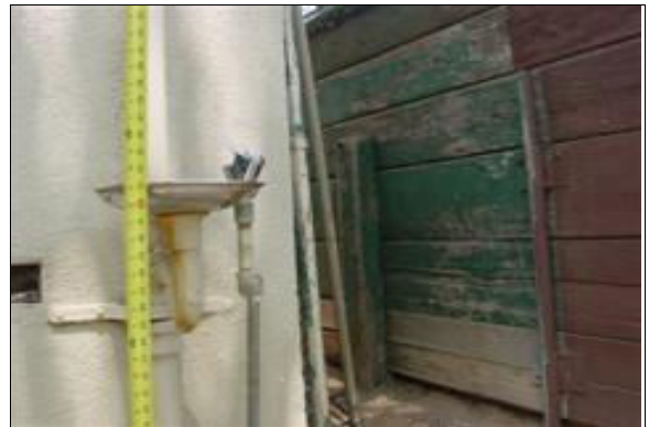
Drinking Fountain Outside of the Press Box (Right)
