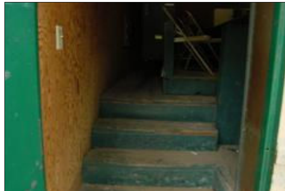
Interior Stairs to the Press Box
