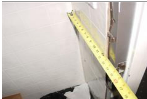
Women's Restroom at the Dad's Club
