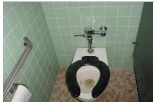
Men's Restroom Across from the Little League Field
