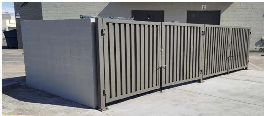
⑱ CMU Block Wall (Angelus Block, Precision, Natural Gray) ⑲ Metal Door (custom fabricated, Metallic Silver)
