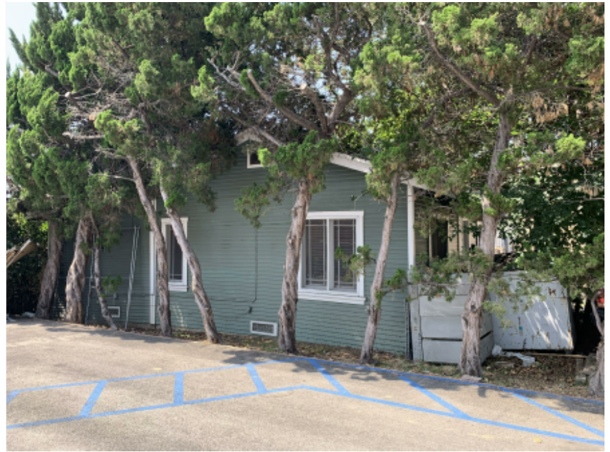
2 SIDE OF RESIDENTIAL BUILDING #1
