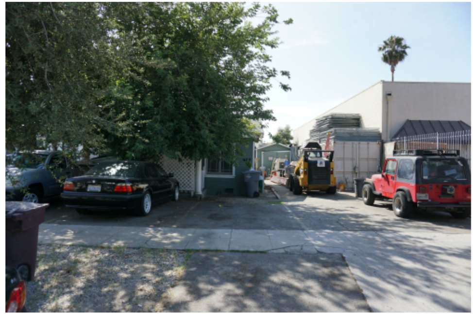
2 FRONT OF PROPERTY
