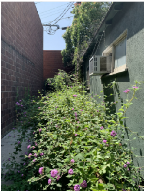
9 SIDE OF RESIDENTIAL BUILDING #2
