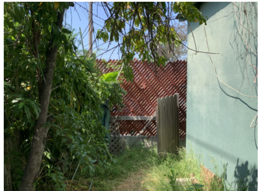
12 REAR OF RESIDENTIAL BUILDING #2
