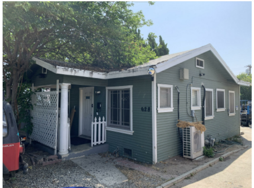
4 SIDE OF RESIDENTIAL BUILDING #1
