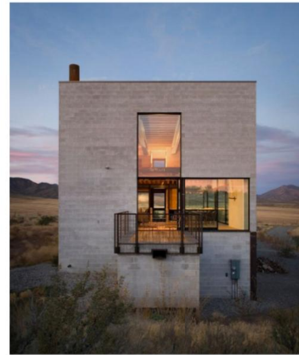
i.e. CMU WALL CONSTRUCTION
