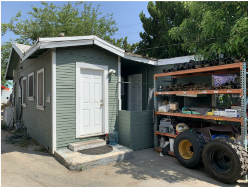
3 REAR OF RESIDENTIAL BUILDING #1
