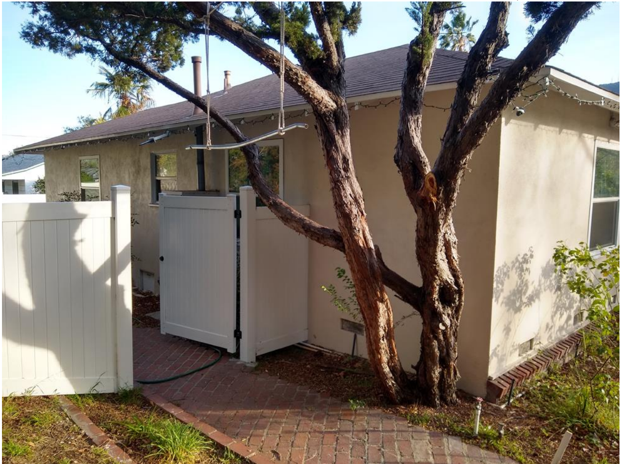
14 – NORTH SIDE OF HOUSE, FROM NORTHWEST CORNER OF PROPERTY
