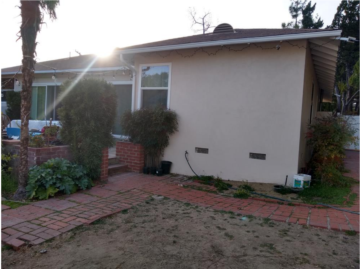
12 - EXISTING EAST WING OF HOUSE, FROM N.E. CORNER OF PROPERTY
