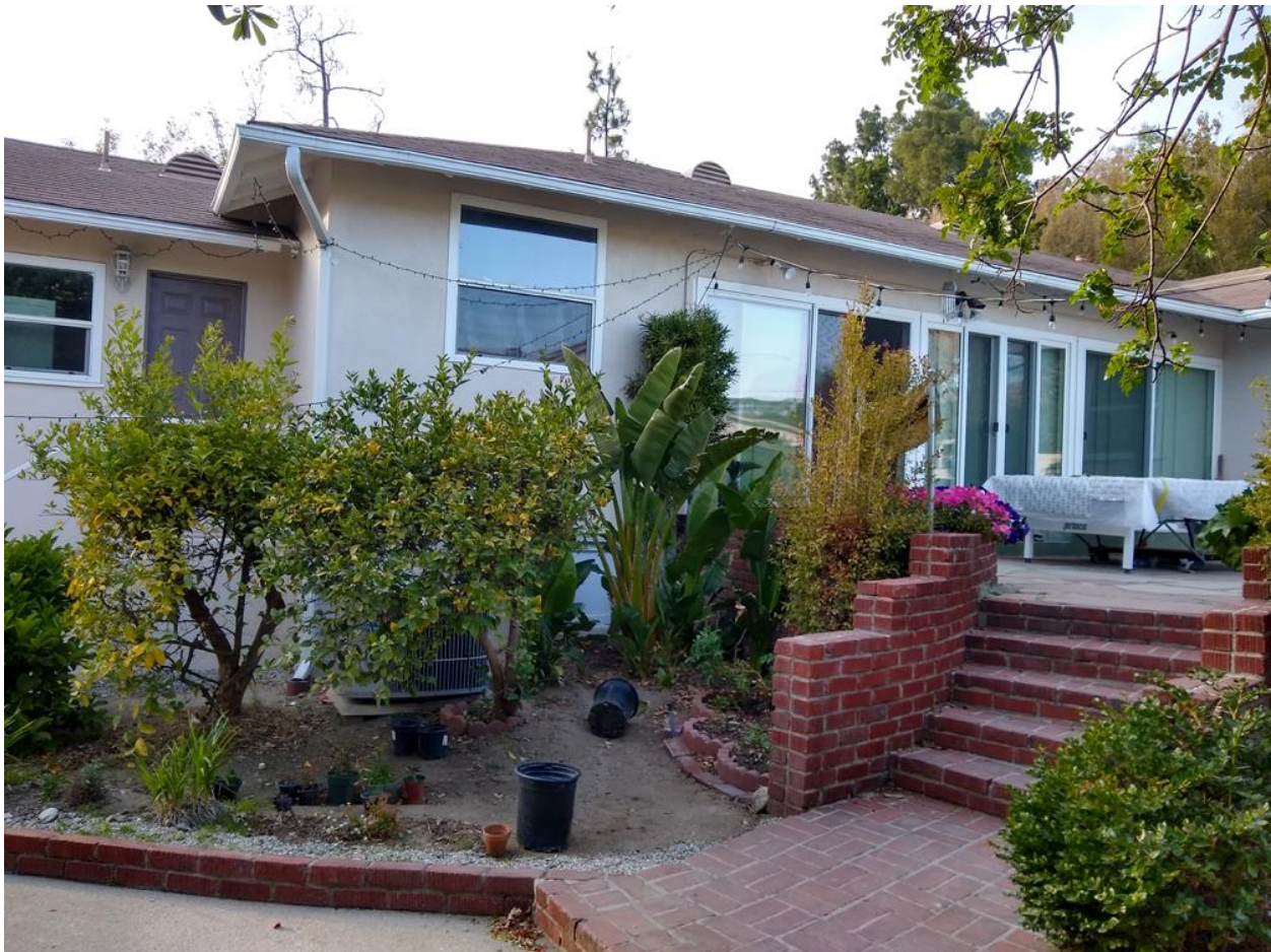
8 – REAR OF HOUSE, FROM BACKYARD
