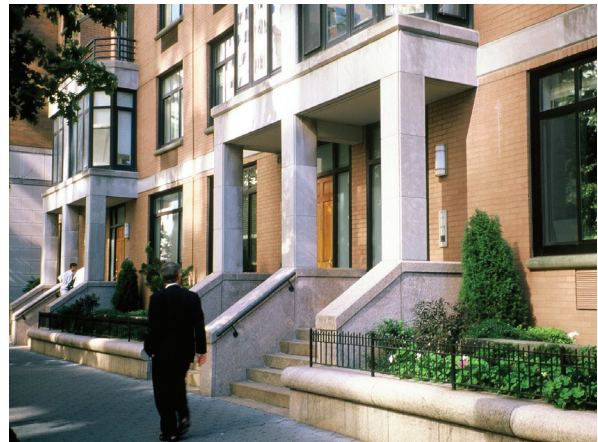
ABOVE: On-street residential entries can increase safety as well as activity on residential-oriented streets.
