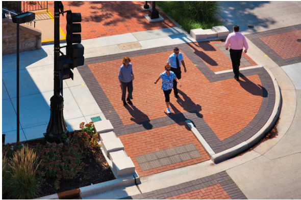
ABOVE: Intersections are important gateways to streets, districts, and significant projects and shall be treated as such with special features such as enhanced paving, and ample room for pedestrian waiting.
