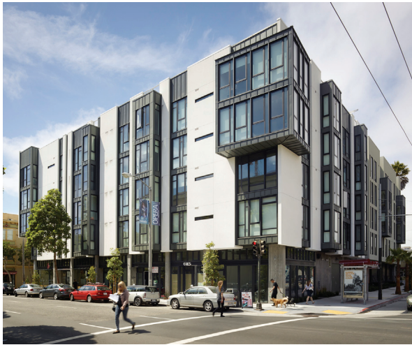
ABOVE: Windows that project out to the street, or recess into the building can create visual interest and depth to a building facade, while also diminishing the scale of the massing.
