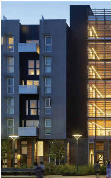
ABOVE: Partially recessed balconies, when combined with major facade modulations can create breaks in large building masses to reduce the overall building scale.
