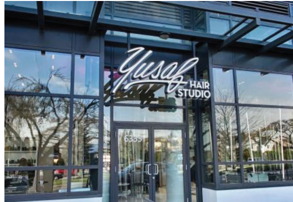
ABOVE: Personalized signage compatible with the architectural character of the building.
