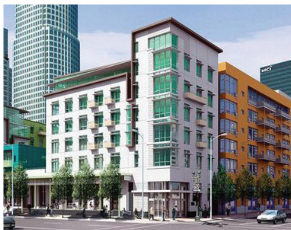
ABOVE: A corner feature can create variation in height while conveying visual prominence for significant intersections or gateways.
