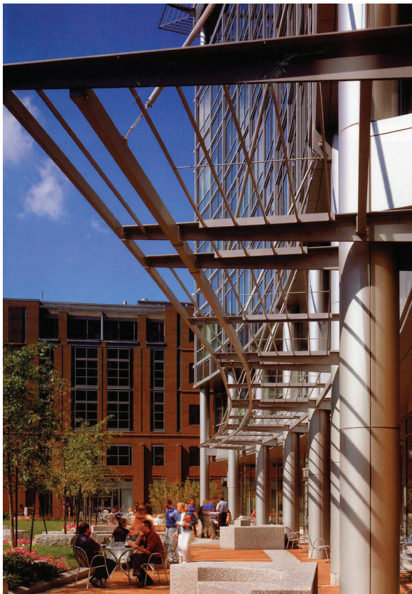
ABOVE: Canopies can serve as sun shading devices, or decorative features that create human-scaled frontages.
