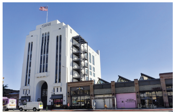
BELOW: In 2016, a full restoration and adaptive reuse of the structure was completed.
