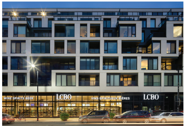
ABOVE: Recessed balconies can be incorporated into a facade design to create a unique pattern or form.
