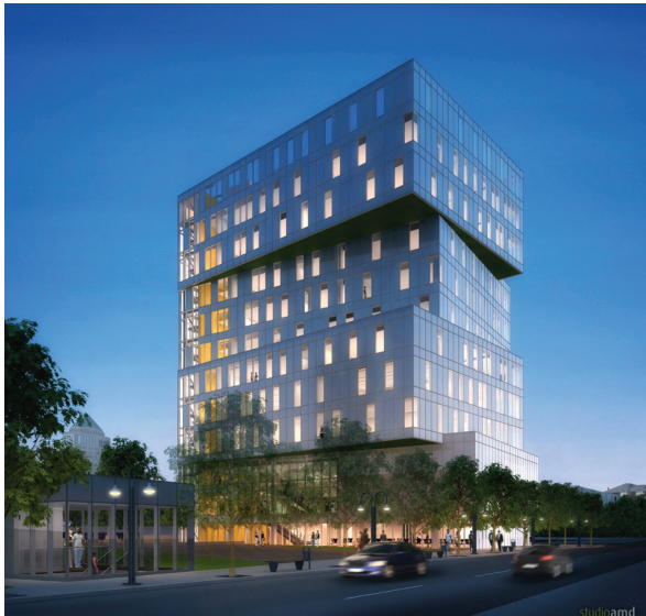
ABOVE: Fenestration patterns that change and respond to form and orientation can enhance modestly designed or flat facades.
