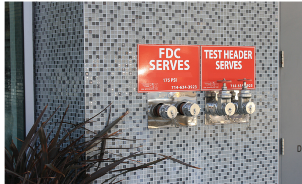
ABOVE: Utilities such as standpipes, fire department connections, and utility boxes are essential to building operations. Utilities shall be incorporated into the building design to the greatest extent feasible, including wall mounted devices, to avoid freestanding obstructions in or near the right-of-way, or visual clutter within landscaped areas or setbacks.
