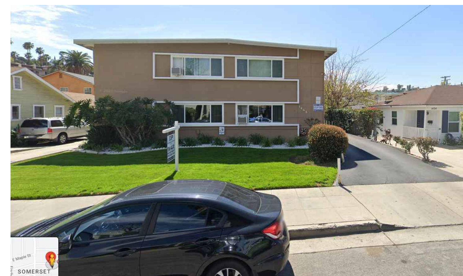
ADJACENT RESIDENTIAL EAST
