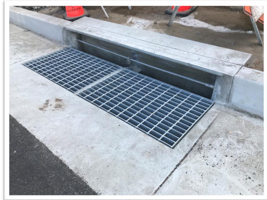
Drywell Installation on Broadway (2022)
