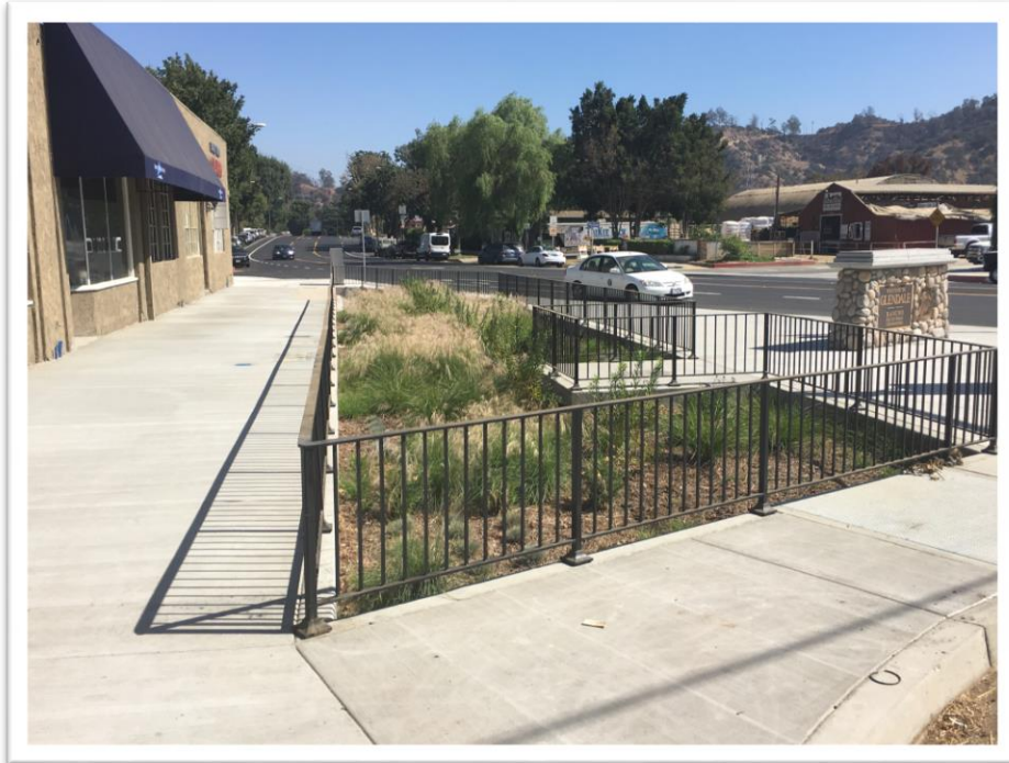
Bioretention Installation at Riverside Drive and Chavez Street (2018)
