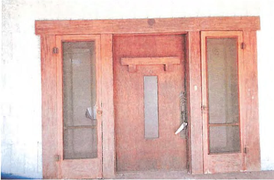
Photograph 2: Detail of natural wood, three-part entry door, screens, doorbell and original, custom hardware. May 2019.
