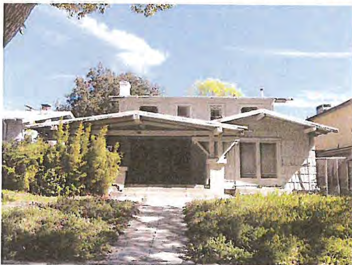
P5a. Photograph or Drawing (Photograph required for buildings, structure, and objects.)
