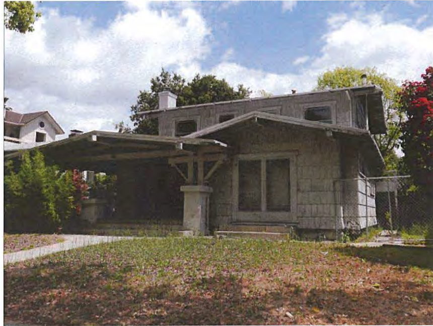
Figure 1B. Primary Façade, 534 N. Kenwood Street SOURCE: Sapphos Environmental, Inc., 2017
