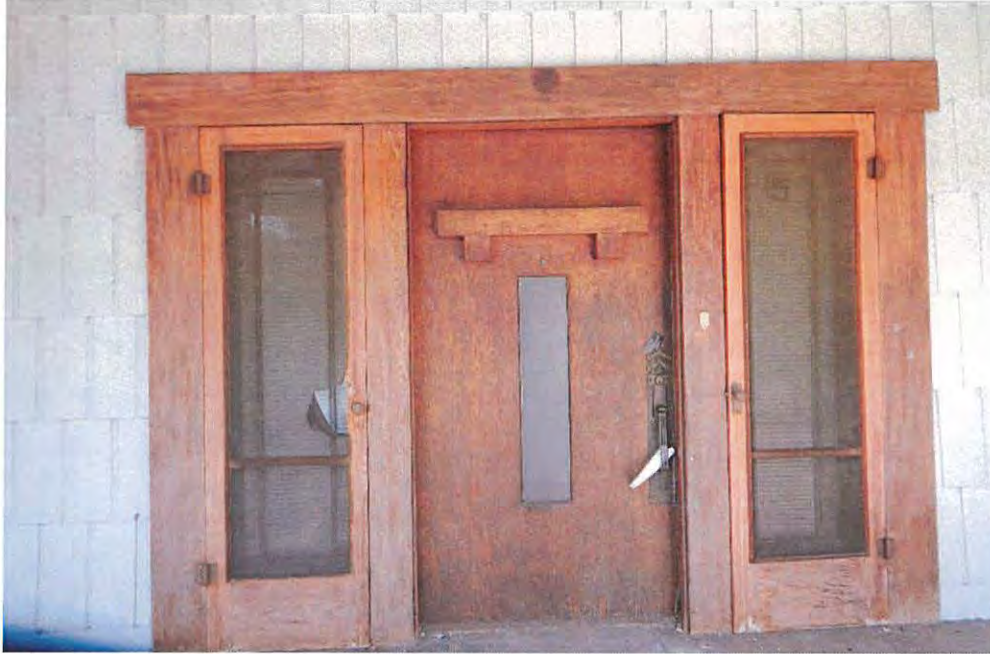
Photograph 2: Detail of natural wood, three-part entry door, screens, doorbell and original, custom hardware. May 2019.
