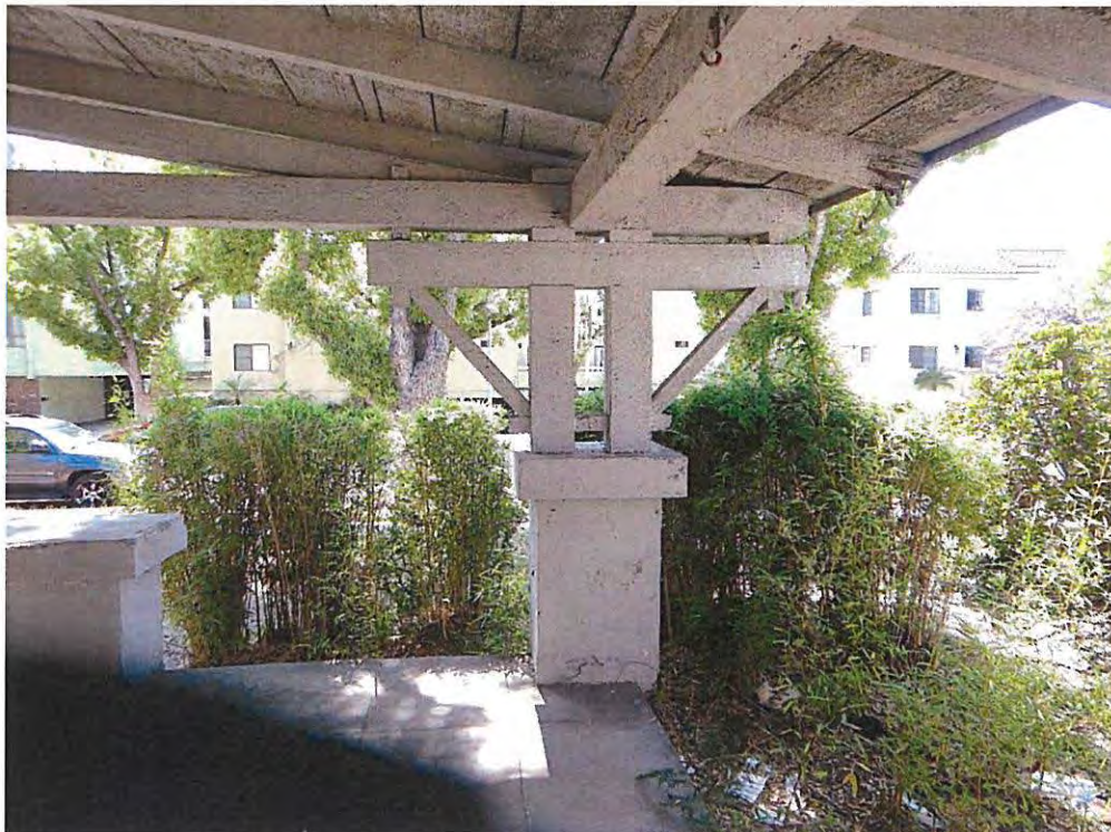
Photograph 3: Detail of double kneebraces, pegged joinery, massive purlin (center top) and open truss (left side) at front porch. May 2019.
