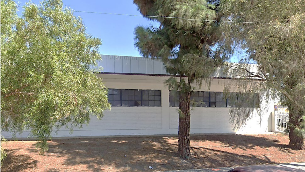
Figure 5: View east of main Hollywood Water Heater Building from San Fernando Road, dated Sept 2022. Source: Google Maps at https://www.google.com/maps/@34.1517383,-118.274298,3a,75y,78.73h,91.84t/data=!3m7!1e1!3m5!1sfhuS0ZRdOorW6WbmWxqtQw!2e0!5s20220901T000000!7i16384!8i8192?hl=en-US
