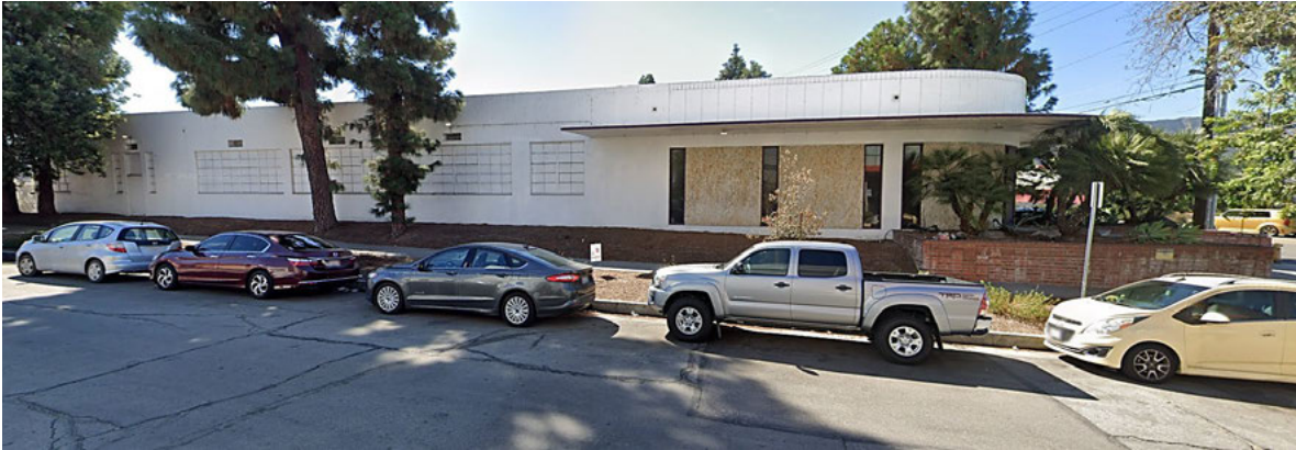
Figure 4: View southeast of Main Building of Hollywood Water Heater Co. from Milford Street, dated Sept 2022. Source: Google Maps at
