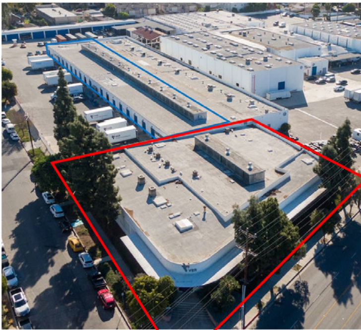
Figure 3: Annotated aerial photograph of Hollywood Water Heater Co. Main Building (outlined in red) and Shipping Building (original exterior demising walls approximately outlined in blue). View southeast. Source: Loop net at https://www.loopnet.com/Listing/5426-5430-San-Fernando-Rd-Glendale-CA/22904260/
