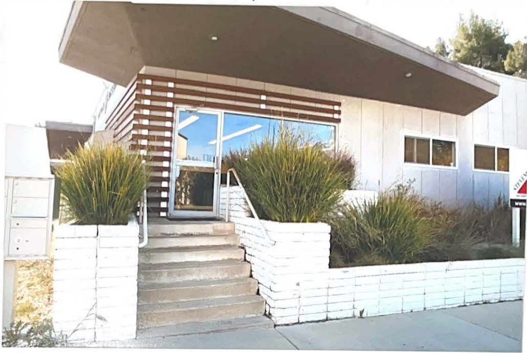
- Stairs (right from the front) entrance 2
