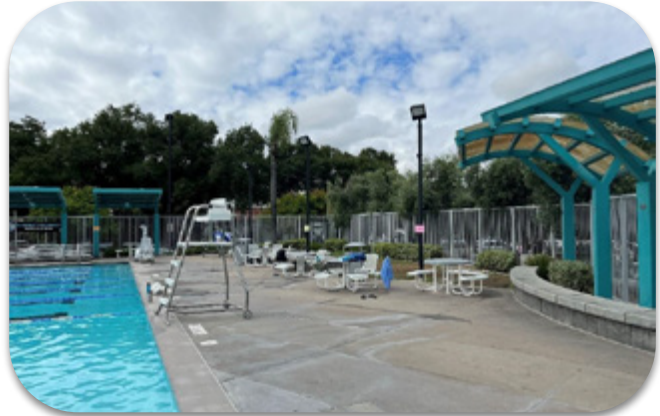
Pacific Community Pool Replaster & Deck
