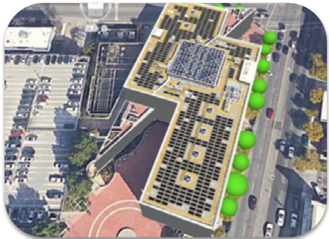
GWP Solar Design Built Program (GWP Perkins Building Rooftop Solar)
