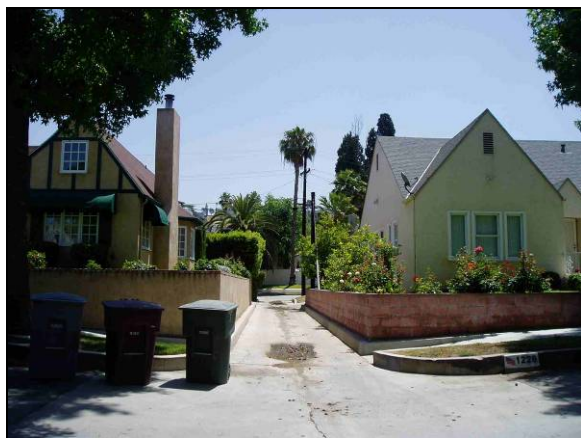
Figure 20 (left) View looking east at the east end of the alley between 1224 and 1228 Cottage Grove Avenue
