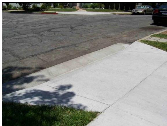
Figure 27 A newer concrete driveway ramp
