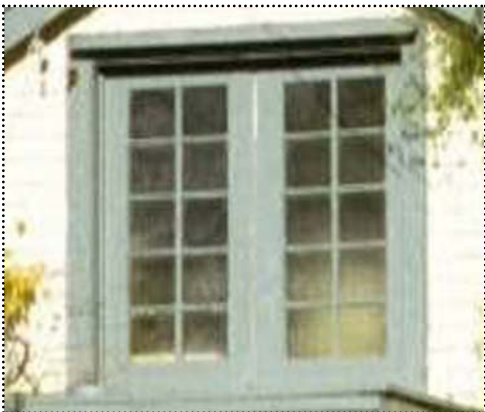
Above: Tripartite wood windows on a Craftsman Below: Wood casement windows
