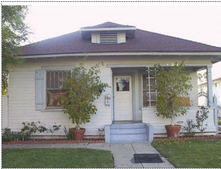
Left: This cottage, built at the turn of the twentieth century, is clad with narrow wooden clapboards.
