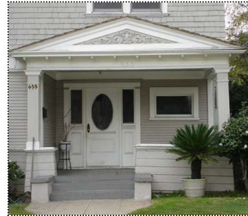
Above: Classically-inspired porch details on this house include a pedimented gable and fluted pilasters with capitals.
