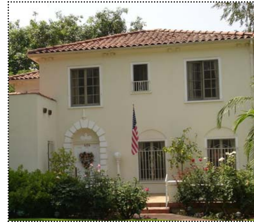
Above: Smooth stucco finish with punched openings are common characteristics.
