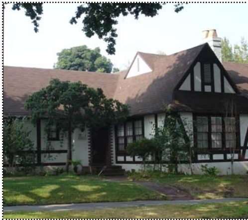
Above: Often Tudor style houses have a variety of roof shapes that break up the massing of the building.
