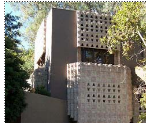
Below: The use of "textile block" in this Lloyd Wright-designed home exhibits an ornamental use of a structural element. Patterned concrete block was used in a similar effect in the Mid-Century Modern houses.
