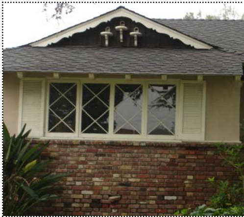
Above: Windows with diamond panes and wood muntins are typical of the style.
