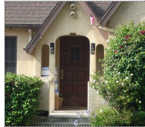
Above: This house has a highly detailed recessed front porch that gives it a great deal of character.
