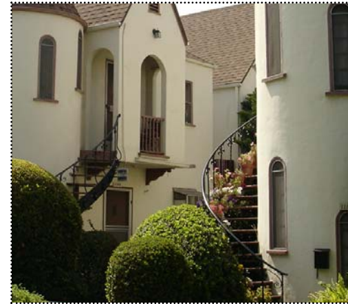
Above: Wrought iron stairs lead to the over-hanging porches on this French eclectic apartment.
