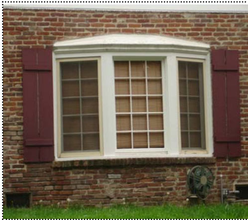
Above: A bay window with shutters is a common element of the Minimal Traditional style.
