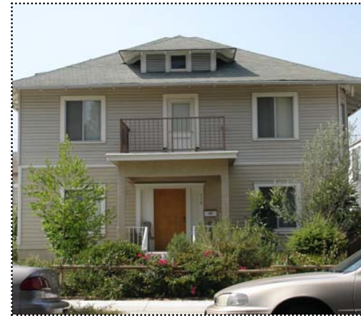
Above: This Foursquare style home in Glendale has narrow wood clapboard siding.
