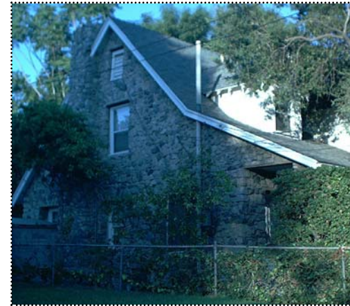
Above: Glendale's stone houses use arroyo stone as the primary exterior finish. These resources are particularly unique and significant among Glendale's rich historic housing stock.
