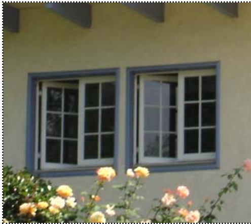
Above: This house has wooden casement windows.
