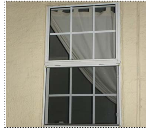
Above: This vinyl window has fake muntins or "grids," which are not appropriate for most historic styles.
