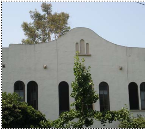
Above: This facade has a roof parapet in the shape of Mission San Antonio de Valero (the Alamo).
