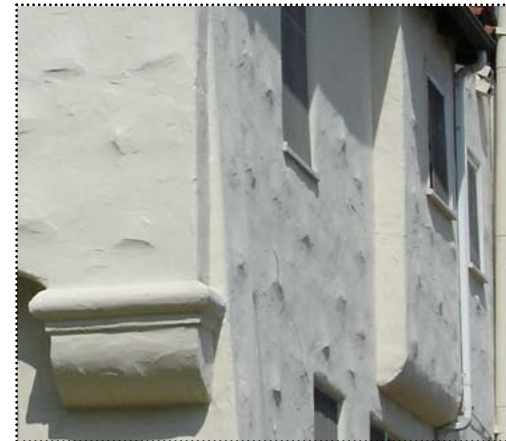
Above: Stucco finish used here is smooth but there are decorative raised areas.
