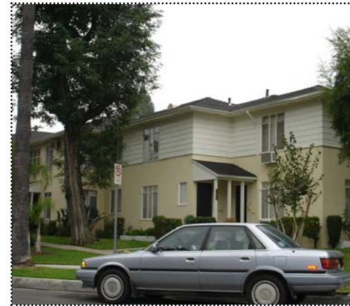
Above: The Minimal Traditional style was used frequently in the design of multi-family houses. This building combines stucco and tongue-in-groove horizontal siding. Its small porticos and limited ornament are also characteristic of the style.
