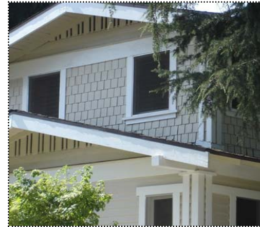
Above: Wood shingles and clapboard siding is most common on Glendale's Craftsman houses.
