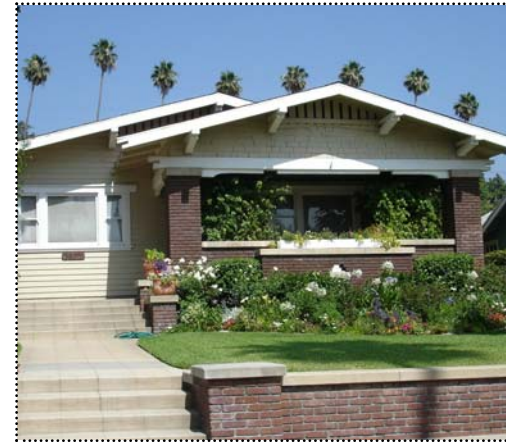
Above: The porch is often a major component of the front of a Craftsman house. Square or battered piers are typically used as porch supports.
