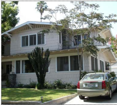
Above: Some Craftsman houses have two stories.
