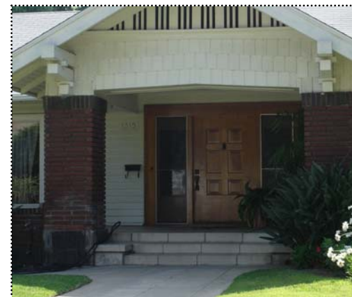
Below: Often the gable end of the porch has the same roofline and materials as the gable of the main house.
