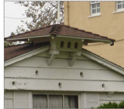
Above: Rooftop cupolas like this one are a common detail of the Ranch style.
