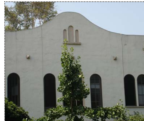
Below: The parapet in this Mission Revival house is a character-defining attribute.
