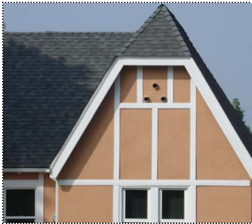
Above: The projecting overhang on this gable and the change in material helps define the character of the house.
