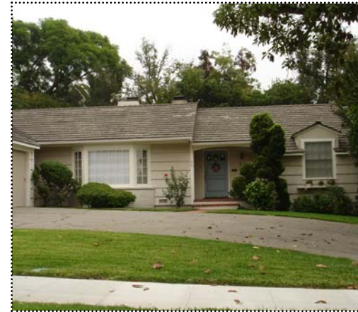
Above: This Ranch house is clad with wide horizontal board siding.
