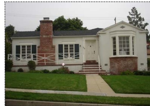
Below: The detailing in this house, shutters and a decorative balustrade, is drawn from the American Colonial Revival.
