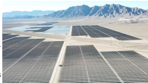
Figure 18. Townsite Solar Plant
