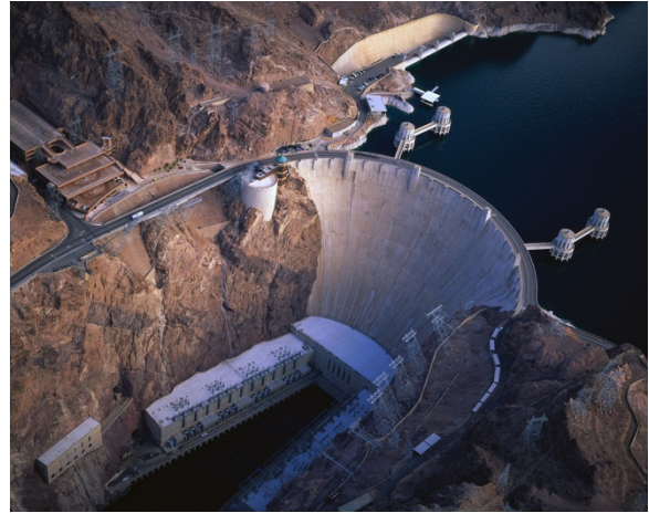
Figure 22. Hoover Dam Power Plant
