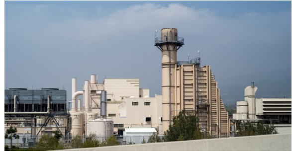
Figure 13. Grayson Power Plant
