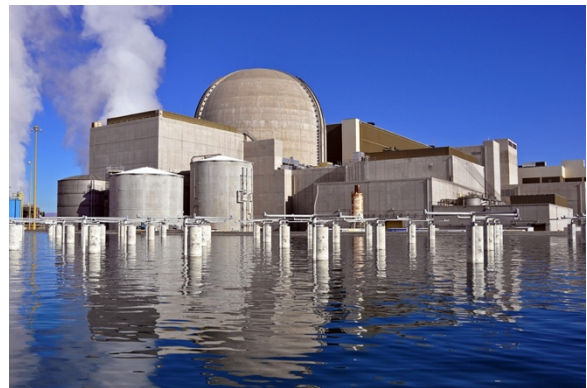
Figure 23. Palo Verde Nuclear Generating Station
