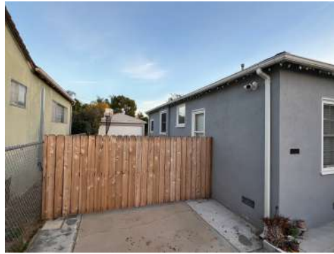
Front Left - South East Facing
