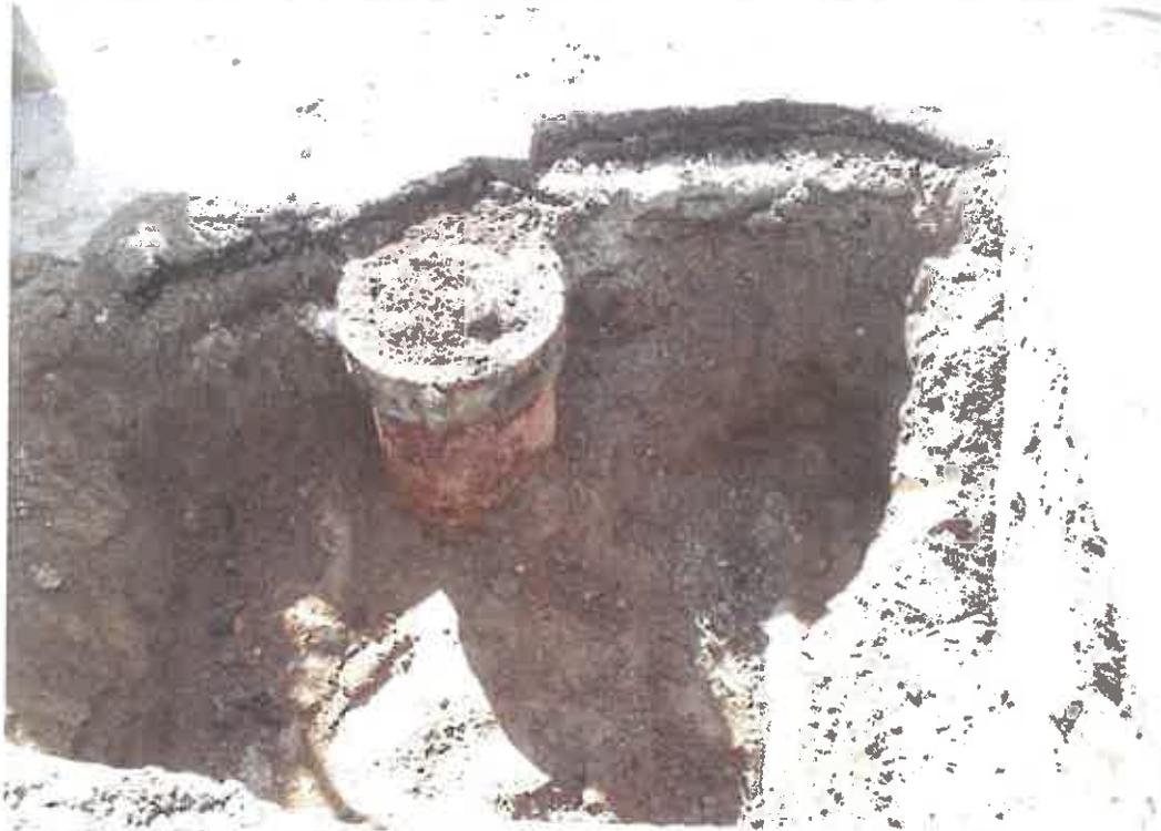
Photograph 17: View of abandoned lift and piping in southern parking area of Site.
