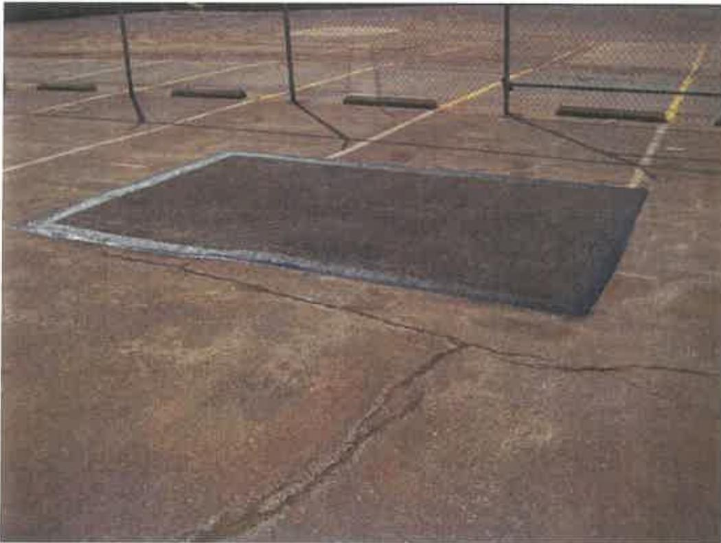
Photograph 18: View of asphalt resurfacing in the location of the former abandoned lift.
