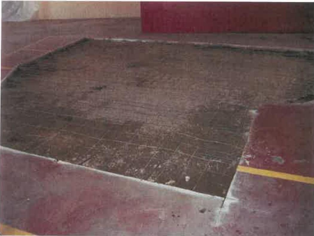
Photograph 10: View of backfilled excavation in Bays 1 and 2 prior to concrete replacement.
