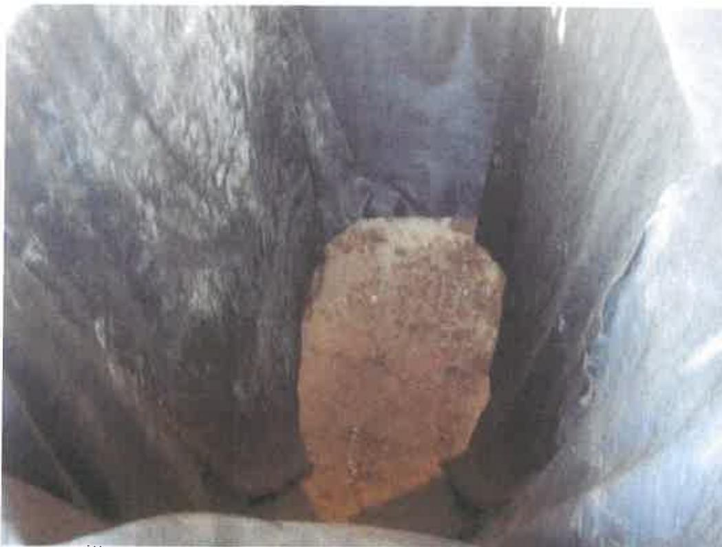
Photograph 8: View of geofabric prior to backfilling excavation.
