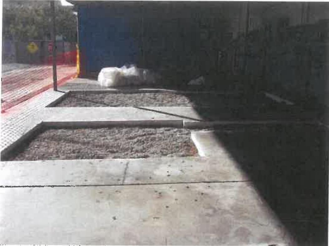
Photograph 9: View of backfilled excavations in Bays 27 and 28 prior to concrete replacement.
