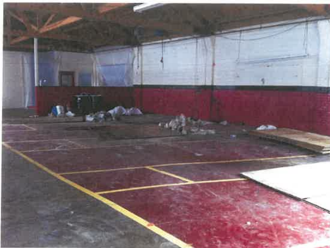
Photograph 1: View of Bays 1 through 4 inside Main Building.
