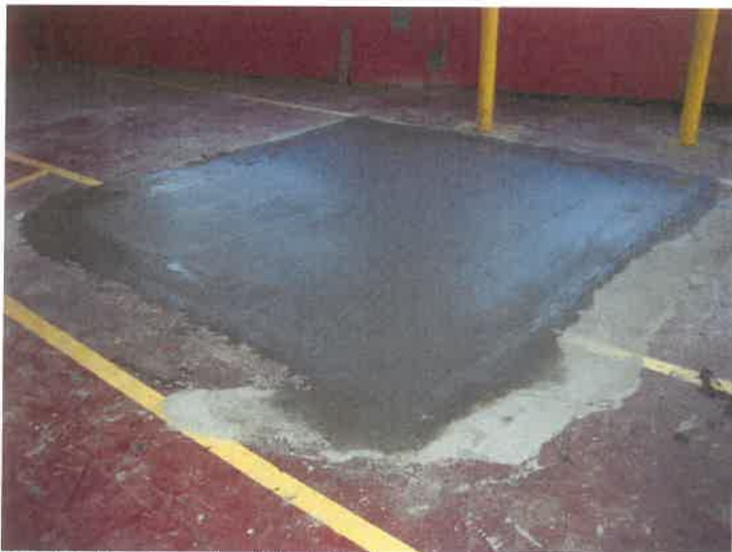
Photograph 8: View of concrete patching in Bay 4.
