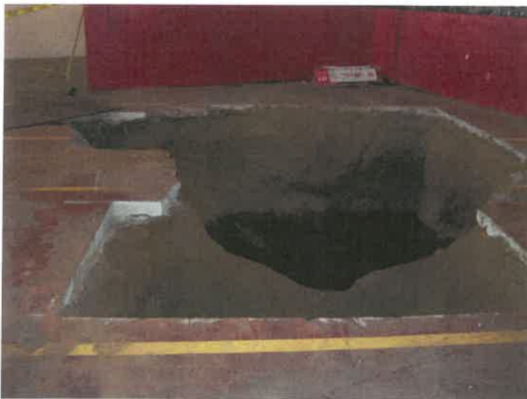
Photograph 2: View of excavation pits in Bays 1 and 2.
