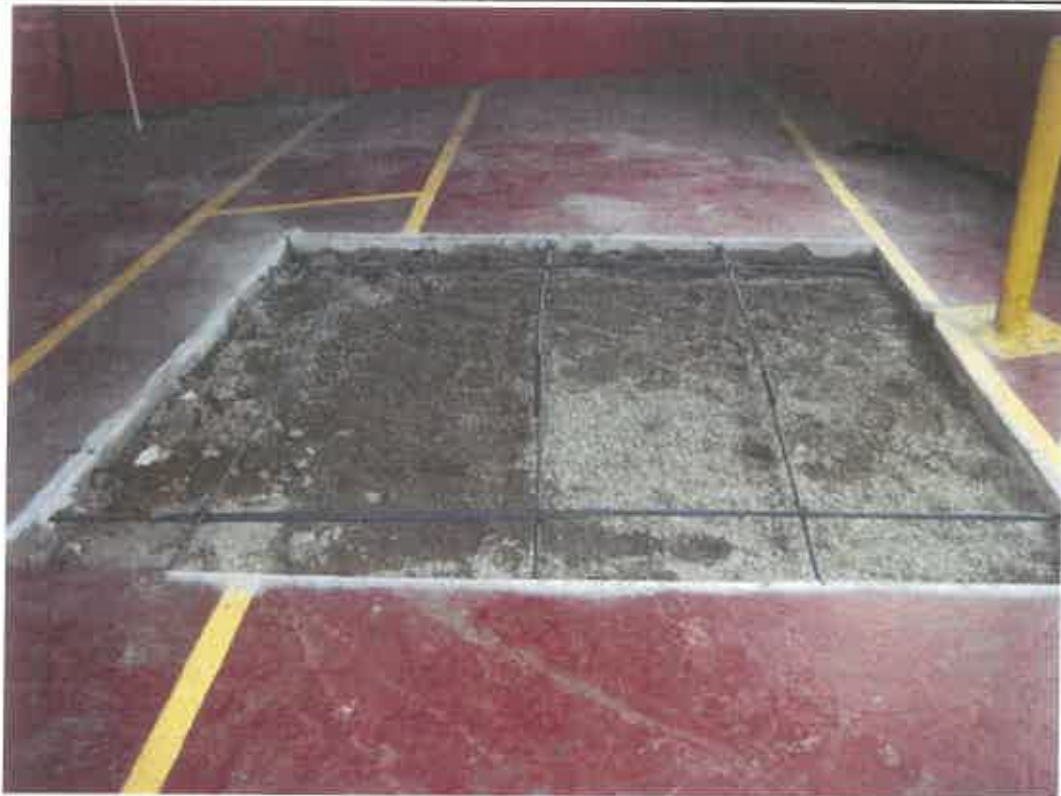
Photograph 7: View of backfilled excavation pit in Bay 4 prior to concrete replacement.
