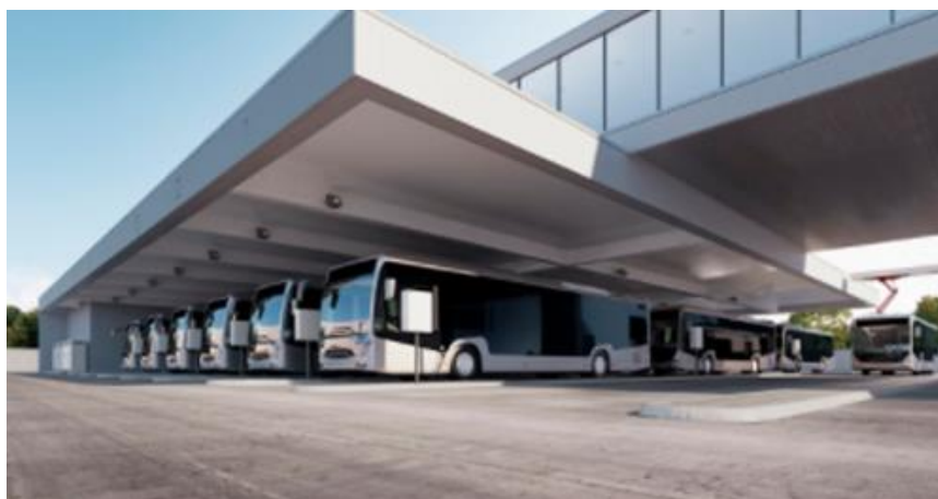
Figure 1-4: Buses Parked in Lanes Example (Source: ABB)
