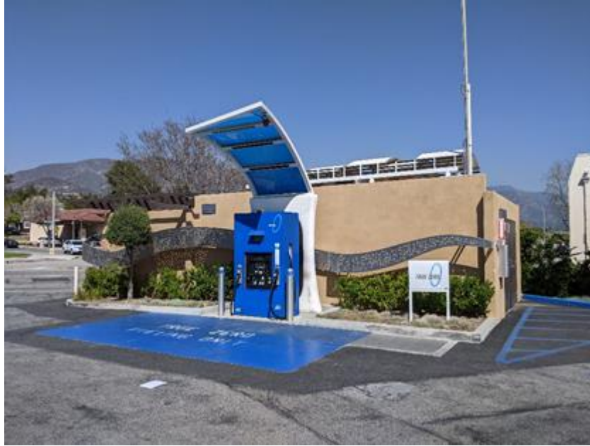
Figure 1-11: True Zero Light-Duty Hydrogen Fueling Station (Source: CALSTART)
