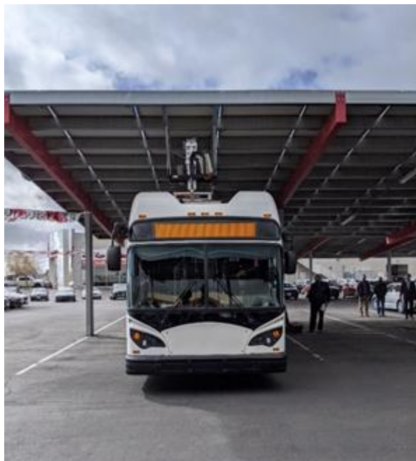
Figure 1-6: In-Depot Overhead Charging Example (Source: CALSTART)
