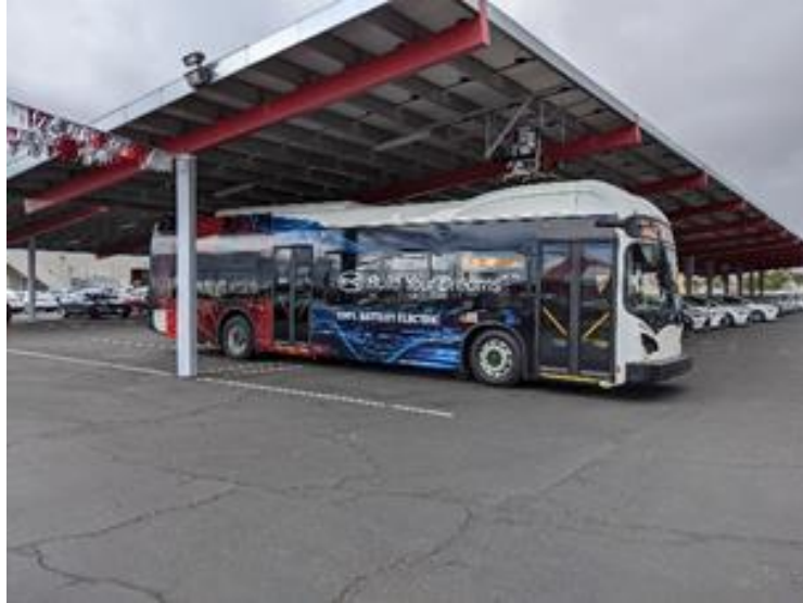
Figure 1-7: In-Depot Overhead Charging Example (Source: CALSTART)
