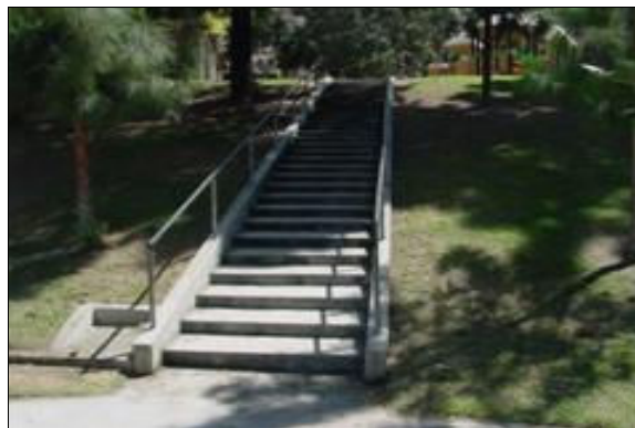
Exterior Stairs to the Lower Play Area
