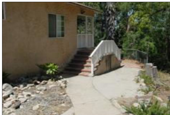
Exterior Stairs at the Caretaker's House
