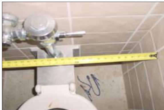
Men's Restroom Next to the Play Equipment Citations: CBC 1115B.7.1.3 ADAAG 4.17.3
