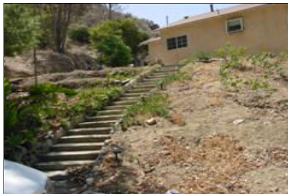
Exterior Stairs to the Caretaker's House
