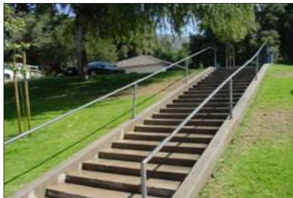
Exterior Stairs to the Baseball Field
