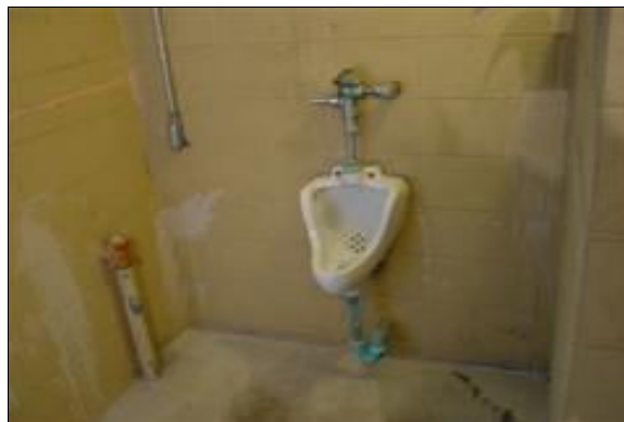
Unisex Restroom at the Maintenance Yard
