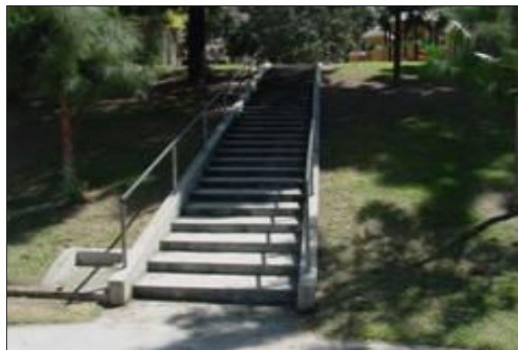
Exterior Stairs to the Lower Play Area
