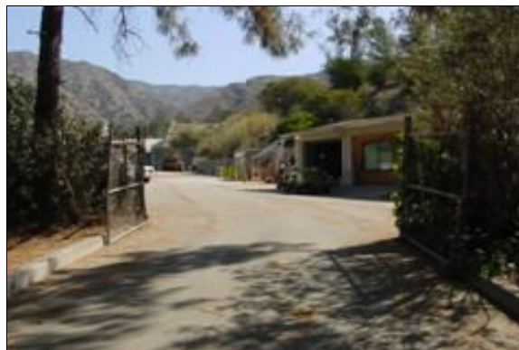
Path of Travel to the Maintenance Yard
