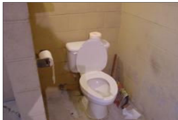
Unisex Restroom at the Maintenance Yard
