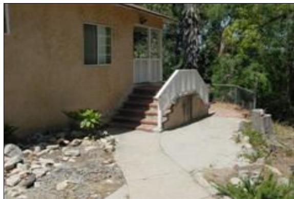
Path of Travel to the Caretaker's House
