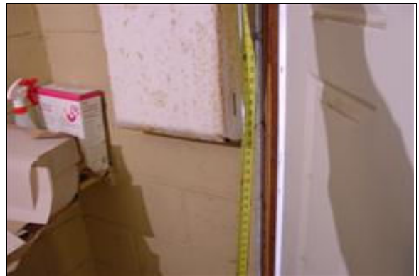
Unisex Restroom at the Maintenance Yard
