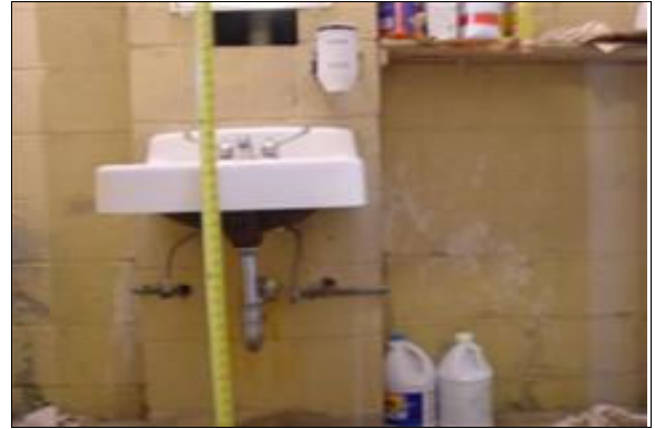
Unisex Restroom at the Maintenance Yard
