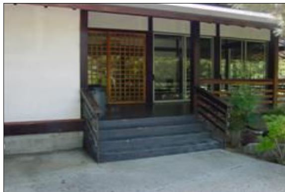
Exterior Stairs to the Tea House
