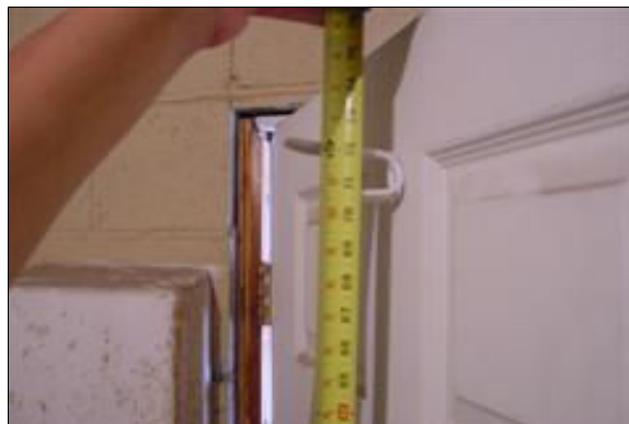
Unisex Restroom at the Maintenance Yard
