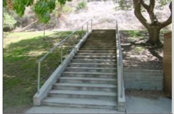
Exterior Stairs at the Restrooms Next to the Play Equipment
