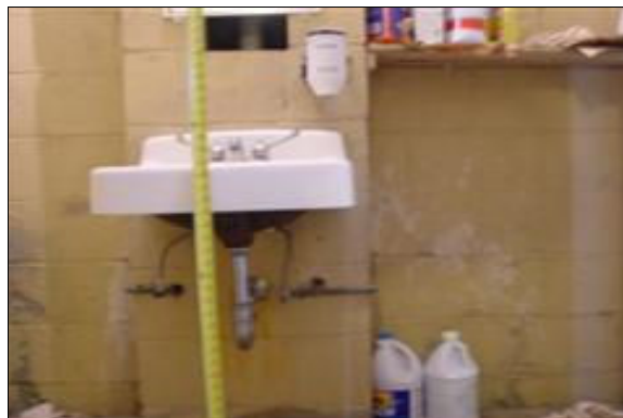
Unisex Restroom at the Maintenance Yard
