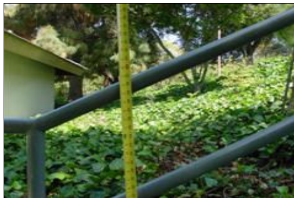
Exterior Stairs to the Upper Parking Lot
