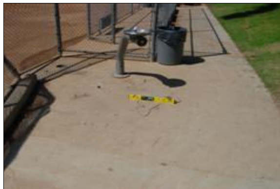
Path of Travel to the Drinking Fountain at the Baseball Field
