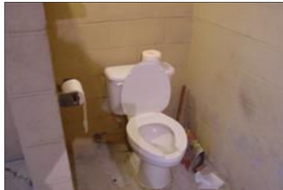
Unisex Restroom at the Maintenance Yard
