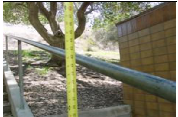
Exterior Stairs at the Restrooms Next to the Play Equipment
