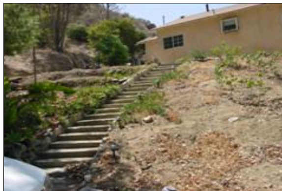
Exterior Stairs to the Caretaker's House
