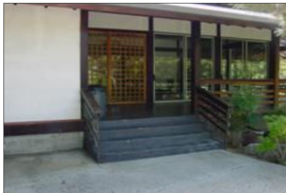
Exterior Stairs to the Tea House
