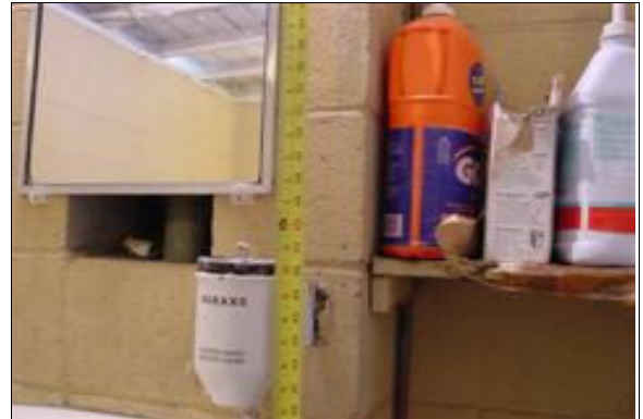
Unisex Restroom at the Maintenance Yard
