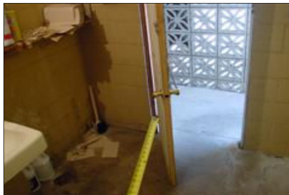
Unisex Restroom at the Maintenance Yard
