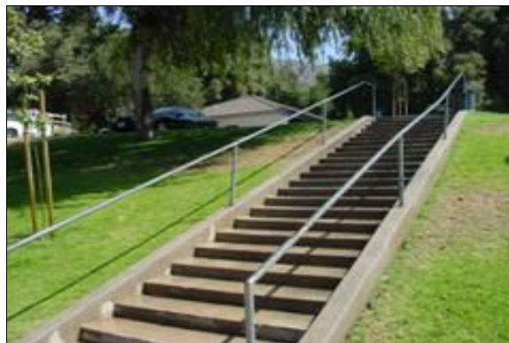
Exterior Stairs to the Baseball Field
