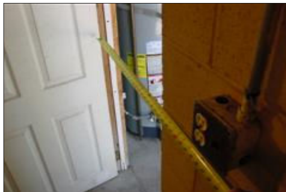
Unisex Restroom at the Maintenance Yard
