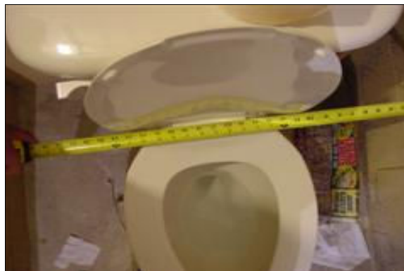
Unisex Restroom at the Maintenance Yard
