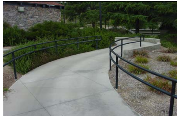
Exterior Ramp to the Restrooms
