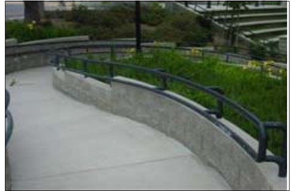
Exterior Ramp Next to the Amphitheater
