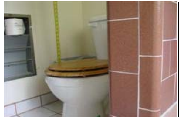
Unisex Restroom in the Ranger Station
