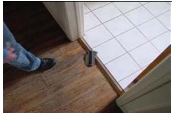
Unisex Restroom in the Ranger Station
