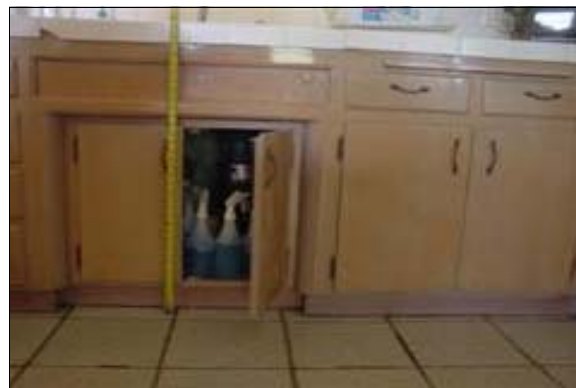
Sink in the Ranger Station
