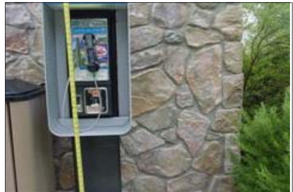
Pay Telephone Next to the Restrooms
