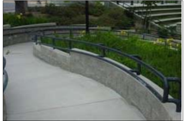
Exterior Ramp Next to the Amphitheater
