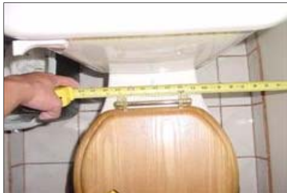
Unisex Restroom in the Ranger Station
