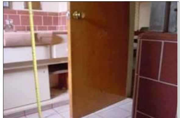
Unisex Restroom in the Ranger Station
