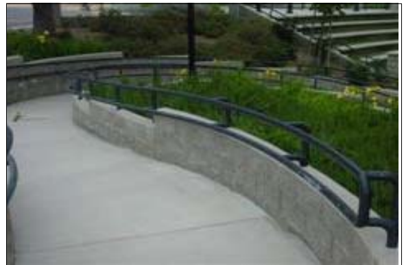
Exterior Ramp Next to the Amphitheater
