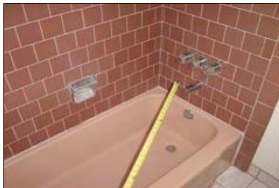
Unisex Restroom in the Ranger Station
