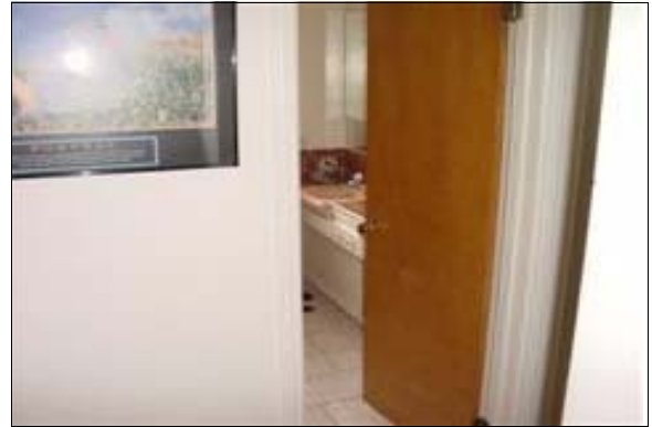
Unisex Restroom in the Ranger Station
