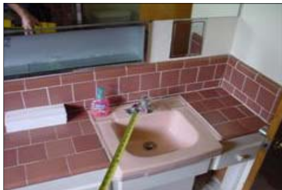
Unisex Restroom in the Ranger Station
