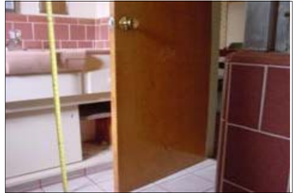
Unisex Restroom in the Ranger Station
