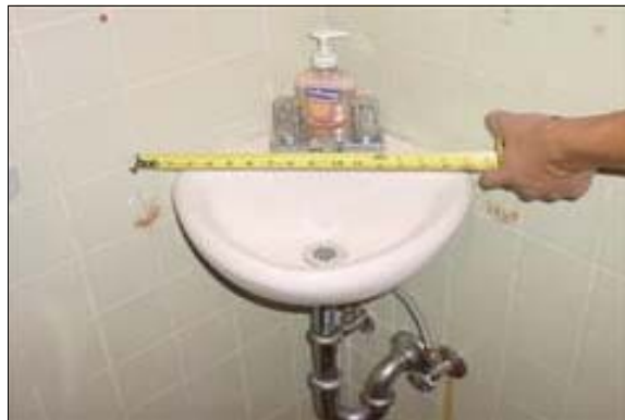
Unisex Restroom in the Community Center
