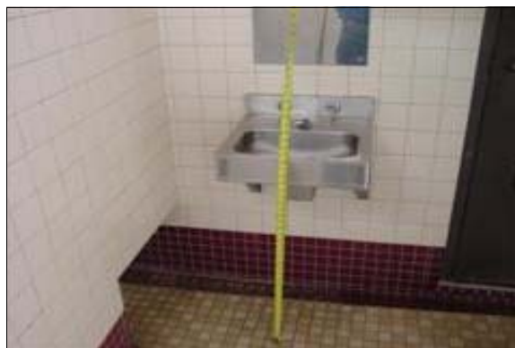
Women's Restroom at the South End of the Park
