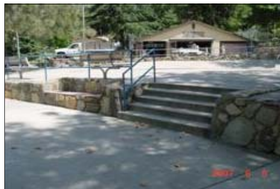
Exterior Stairs to the Wading Pool
