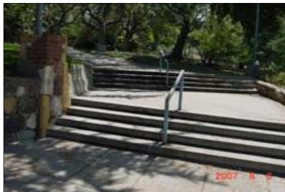
Exterior Stairs at the North End of the Park
