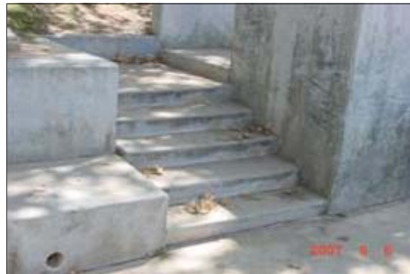
Exterior Stairs to the Press Box at the Baseball Field
