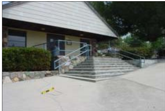
Path of Travel to the Community Center
