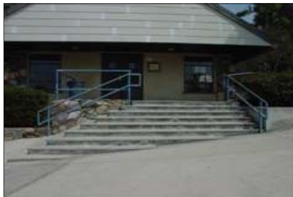
Exterior Stairs to the Community Center
