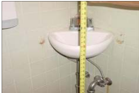
Unisex Restroom in the Community Center
