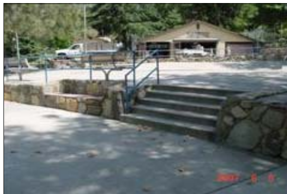
Exterior Stairs to the Wading Pool
