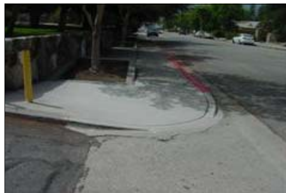
Curb Ramp at the Entrance to the Public Parking Lot (Right)
