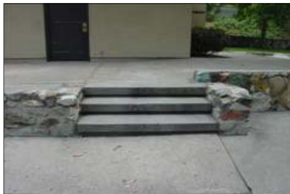
Exterior Stairs to the North Restroom
