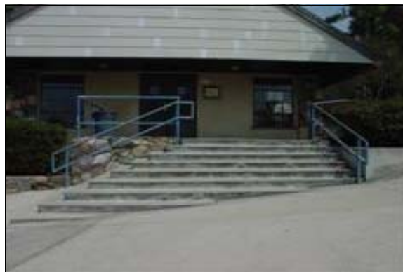
Exterior Stairs to the Community Center
