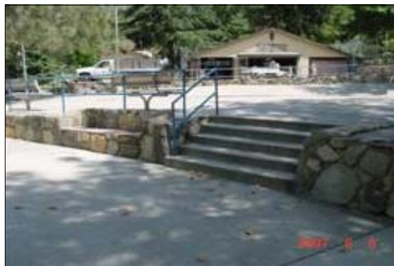
Exterior Stairs to the Wading Pool
