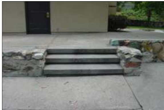
Exterior Stairs to the North Restroom
