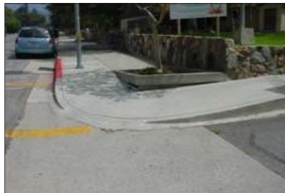
Curb Ramp at the Entrance to the Public Parking Lot (Left)
