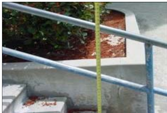
Exterior Stairs to the Community Center
