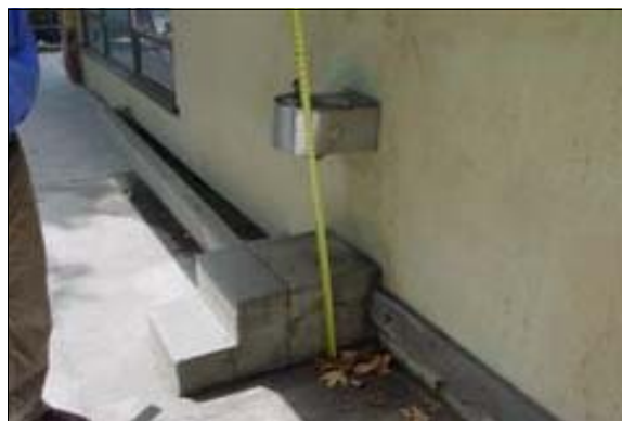
Drinking Fountain Outside of the Community Center
