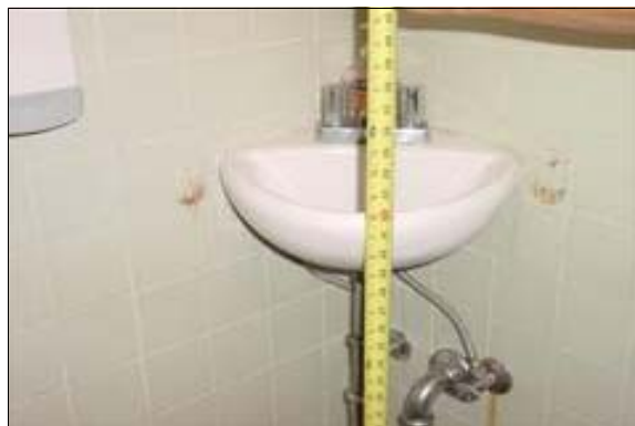
Unisex Restroom in the Community Center
