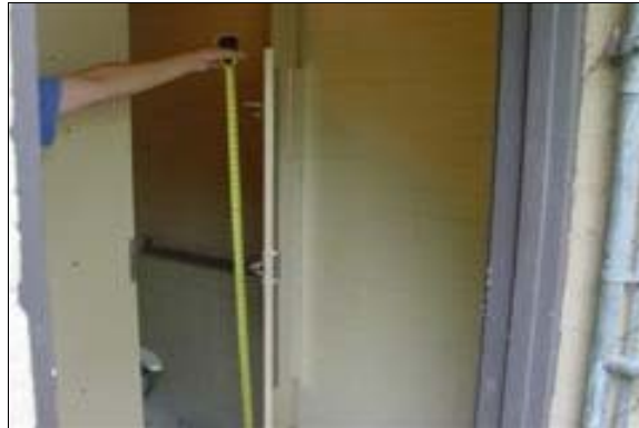
Men's Restroom at the North End of the Park
