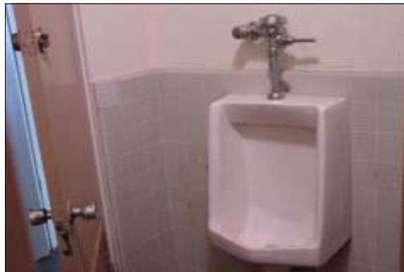
Unisex Restroom in the Community Center
