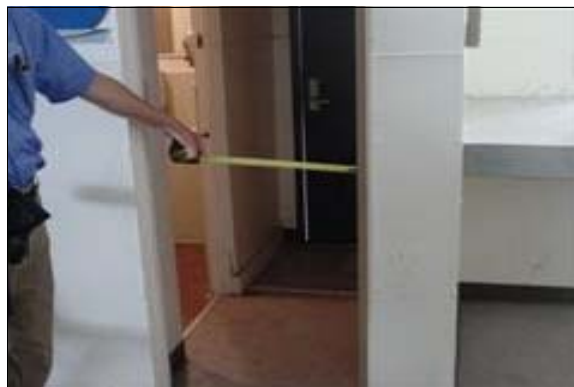
Unisex Restroom in the Community Center
