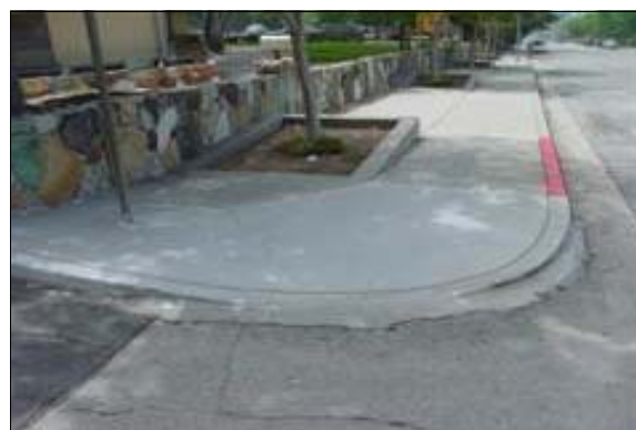
Curb Ramp at the Entrance to the Employee Parking Lot (Right)
