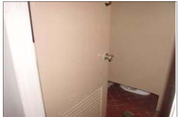
Unisex Restroom in the Community Center
