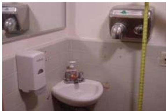
Unisex Restroom in the Community Center
