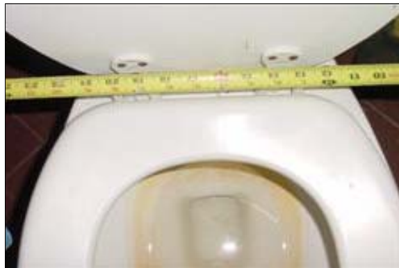
Unisex Restroom in the Community Center
