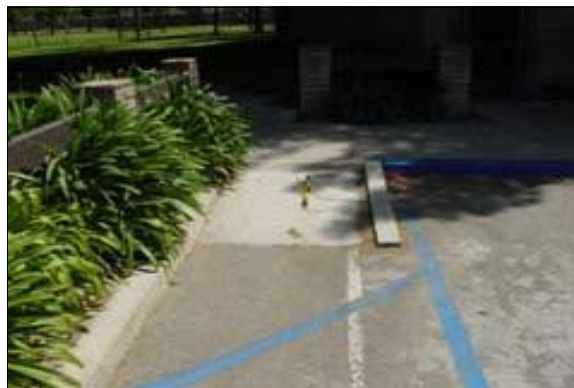
Curb Ramp at the Accessible Parking Space
