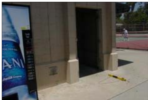
Women's Restroom at the Tennis Courts
