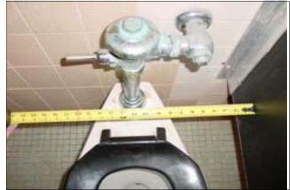
Men's Restroom at the Tennis Courts
