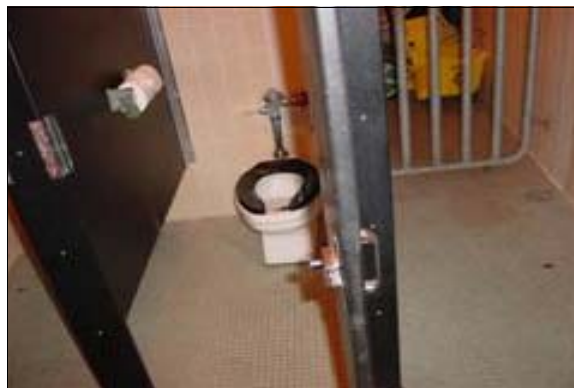
Men's Restroom at the Tennis Courts
