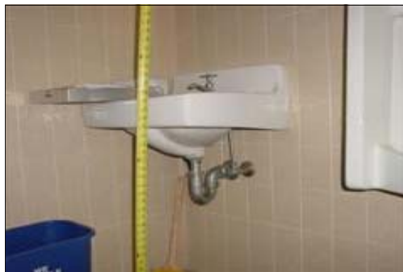
Unisex Restroom at the Maintenance Building
