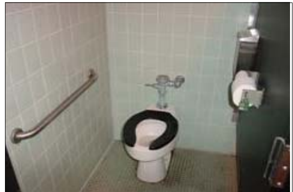
Women's Restroom at the Tennis Courts
