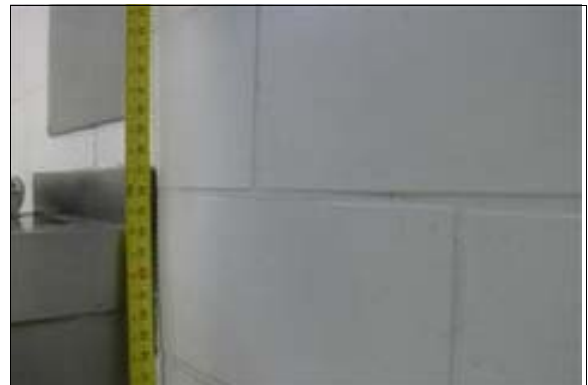
Men's Restroom Next to the Play Equipment
