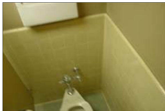
Unisex Restroom at the Maintenance Building
