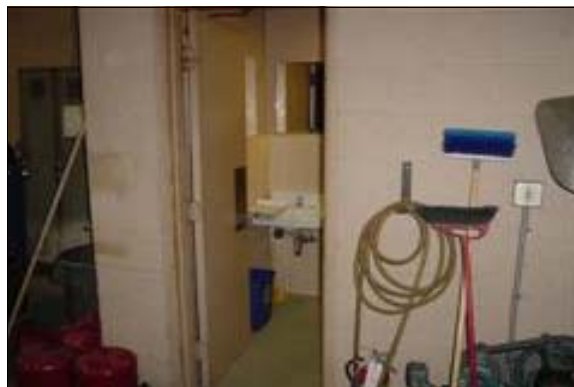
Unisex Restroom at the Maintenance Building
