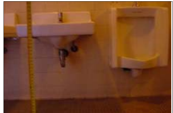
Men's Restroom at the Tennis Courts
