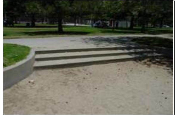
Exterior Stairs to the Play Area
