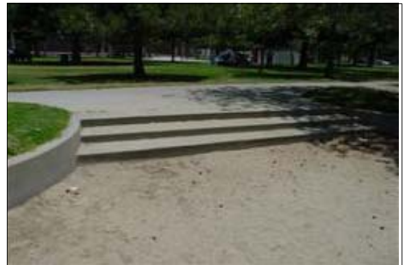
Exterior Stairs to the Play Area
