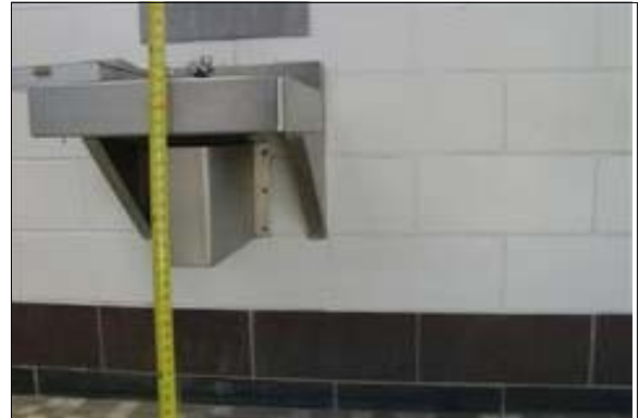
Men's Restroom Next to the Play Equipment
