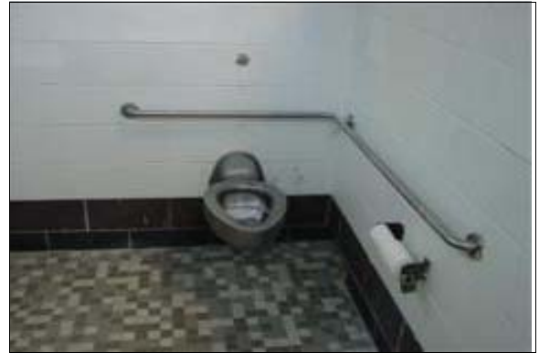
Men's Restroom Next to the Play Equipment
