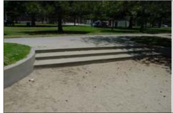
Exterior Stairs to the Play Area
