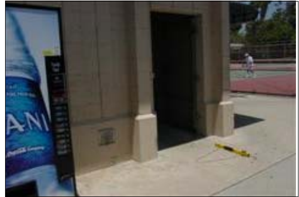
Women's Restroom at the Tennis Courts
