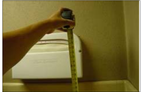
Unisex Restroom at the Maintenance Building
