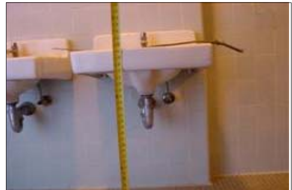
Women's Restroom at the Tennis Courts
