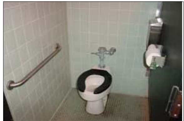
Women's Restroom at the Tennis Courts
