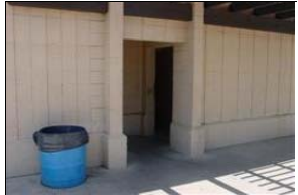
Men's Restroom at the Tennis Courts
