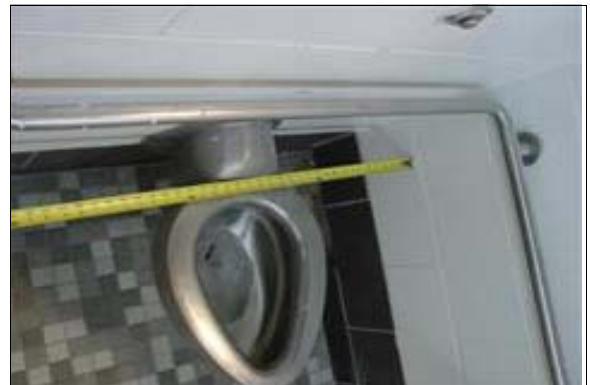
Men's Restroom Next to the Play Equipment
