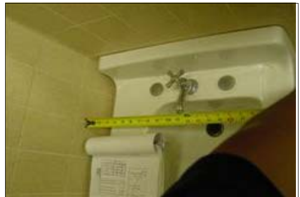
Unisex Restroom at the Maintenance Building
