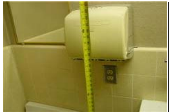
Unisex Restroom at the Maintenance Building
