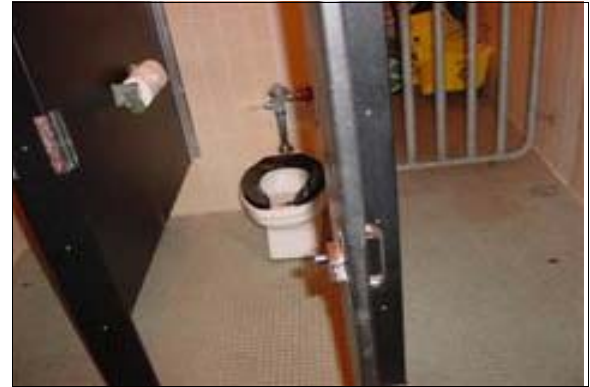
Men's Restroom at the Tennis Courts
