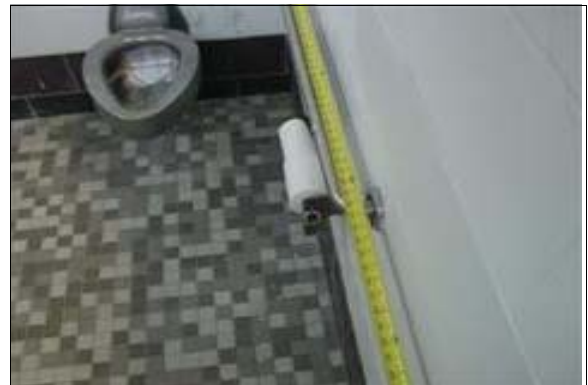
Men's Restroom Next to the Play Equipment
