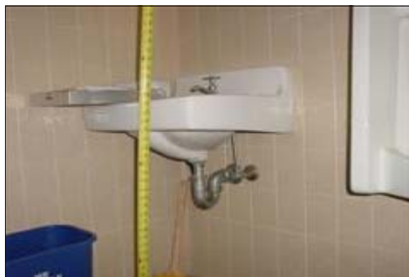
Unisex Restroom at the Maintenance Building
