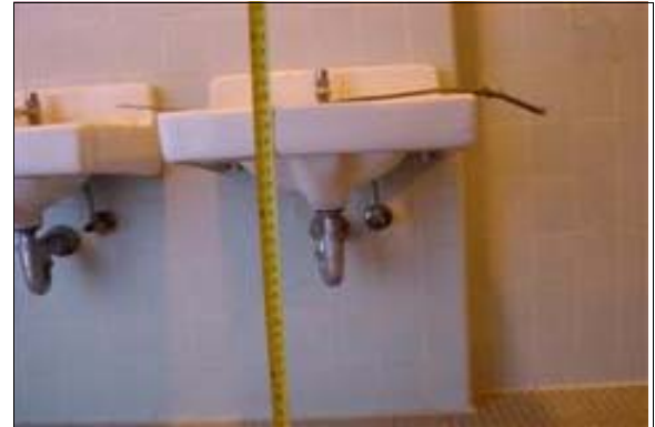
Women's Restroom at the Tennis Courts
