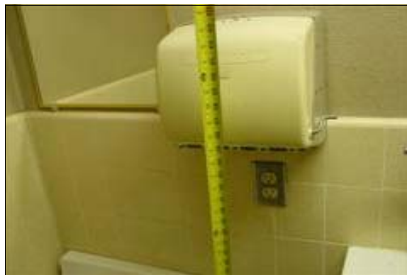
Unisex Restroom at the Maintenance Building
