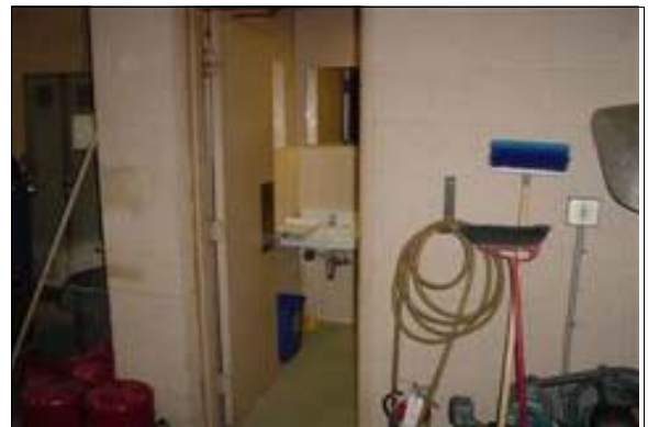
Unisex Restroom at the Maintenance Building
