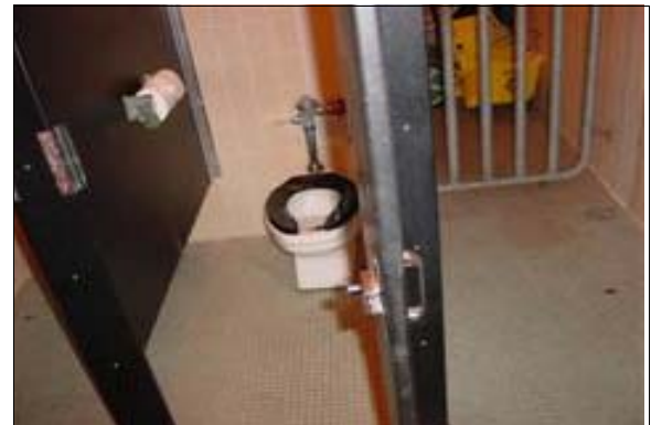
Men's Restroom at the Tennis Courts
