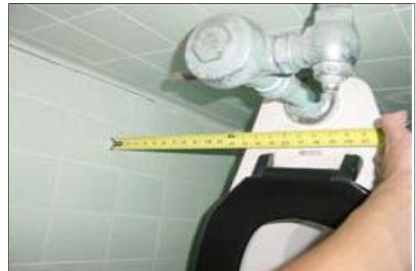
Women's Restroom at the Tennis Courts
