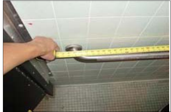
Women's Restroom at the Tennis Courts
