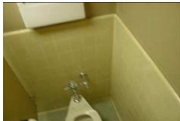
Unisex Restroom at the Maintenance Building
