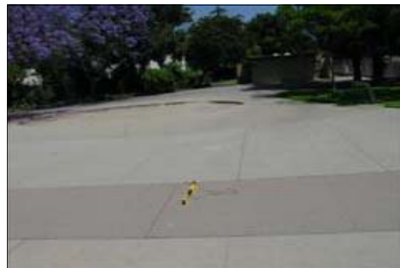
Path of Travel to the Restrooms
