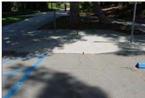
Curb Ramp at the Accessible Parking Space
