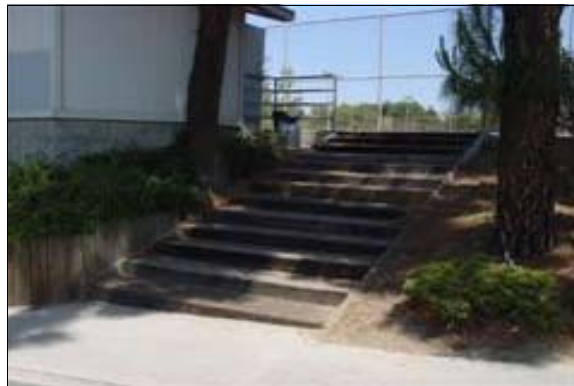
Exterior Stairs to the Tennis Courts
