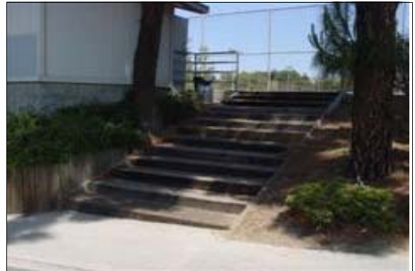
Exterior Stairs to the Tennis Courts
