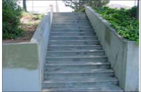
Exterior Stairs to the Tennis Courts
