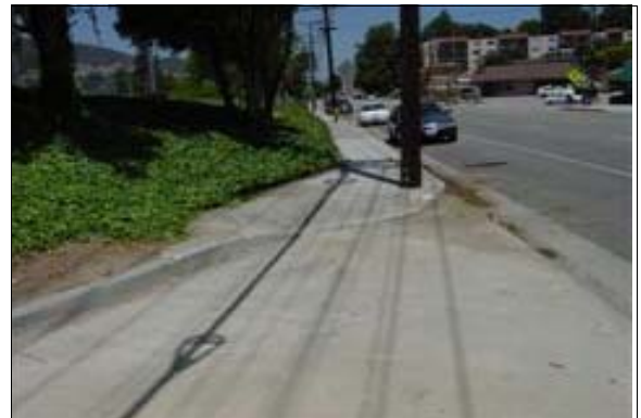
Curb Ramp off of Verdugo (Right)
