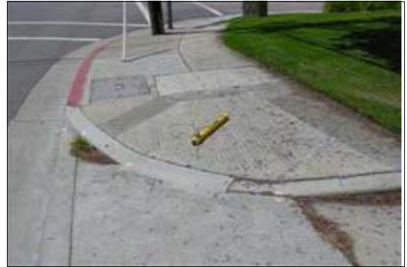
Curb Ramp off of Verdugo (Left)
