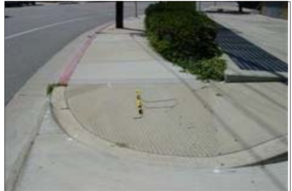
Curb Ramp off of Verdugo (Center Right)
