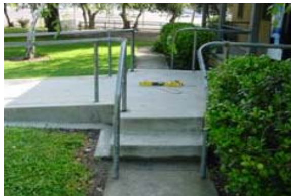
Exterior Stairs to the Community Center
