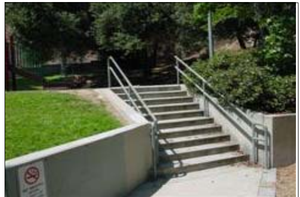
Exterior Stairs to the Play Equipment (Right)
