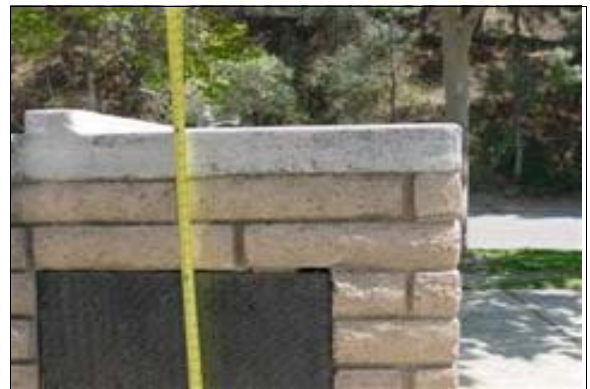
Sink at the Outdoor Dining Area
