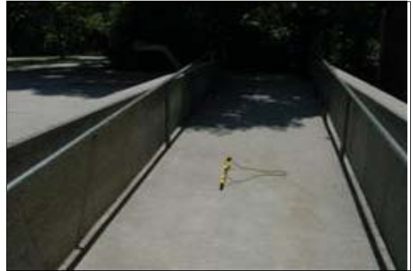
Exterior Ramp Next to the Restrooms
