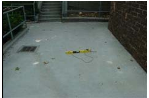
Path of Travel Between the Men's and Women's Restrooms
