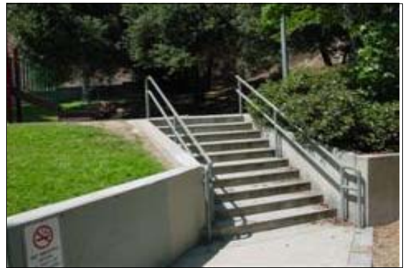
Exterior Stairs to the Play Equipment (Right)
