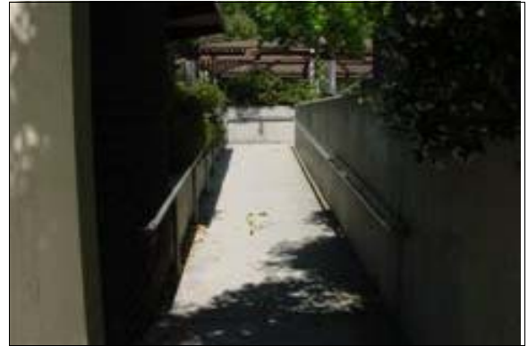
Exterior Ramp Next to the Restrooms
