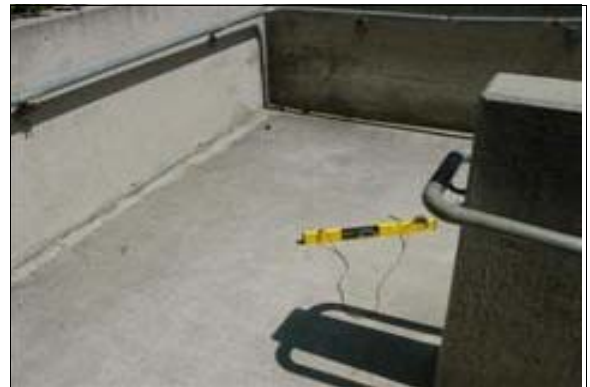
Exterior Ramp Next to the Restrooms
