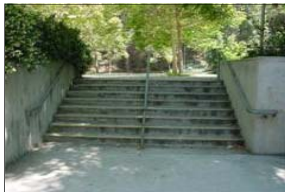
Exterior Stairs to the Lower Outdoor Dining Area (South)
