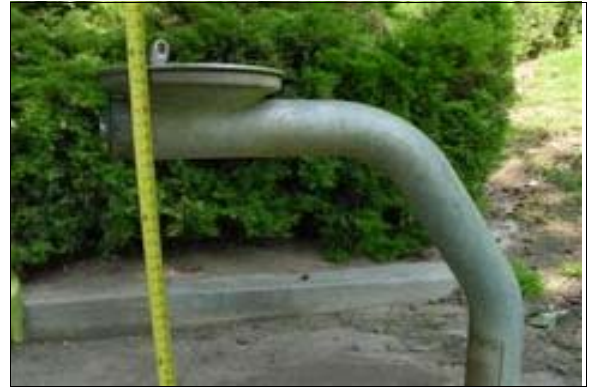
Drinking Fountain at the Lower Outdoor Dining Area
