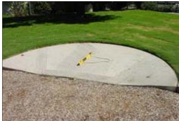
Curb Ramp at the Play Equipment
