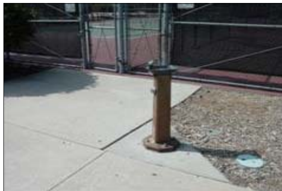
Drinking Fountain at the Tennis Courts
