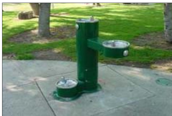
Drinking Fountain at the Restrooms
