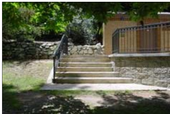
Exterior Stairs to the Restrooms
