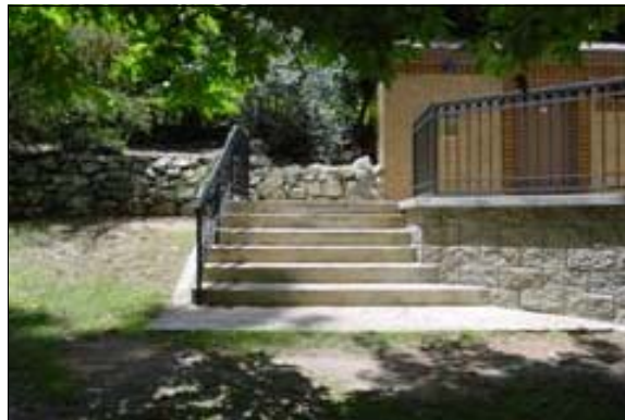
Exterior Stairs to the Restrooms
