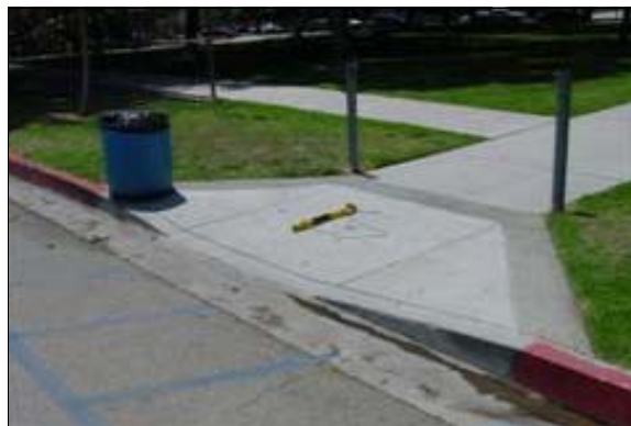
Curb Ramp Next to the Accessible Parking Space
