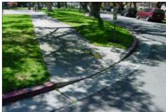
Curb Ramp (West)
