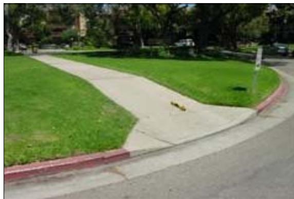
Curb Ramp (South)
