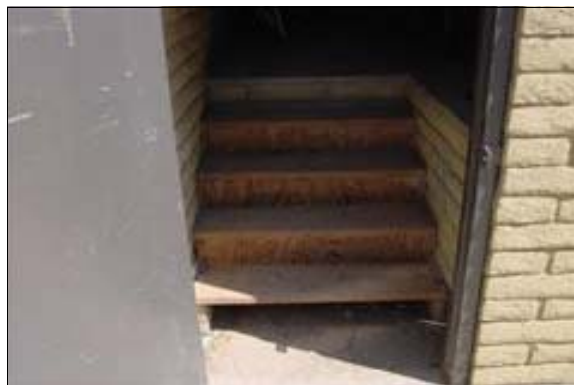
Exterior Stairs to Press Box 3
