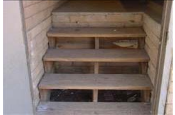
Exterior Stairs to Press Box 1
