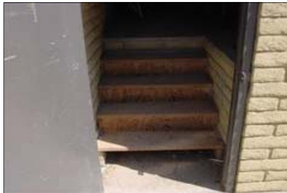
Exterior Stairs to Press Box 3
