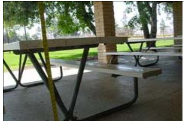
Outdoor Dining Area Next to the Maintenance Building
