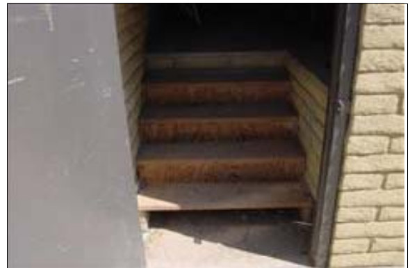
Exterior Stairs to Press Box 3
