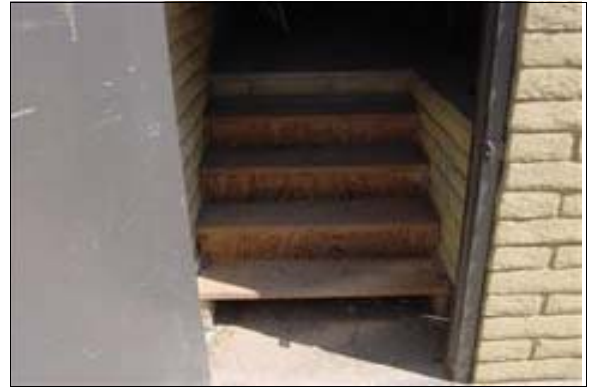
Exterior Stairs to Press Box 3
