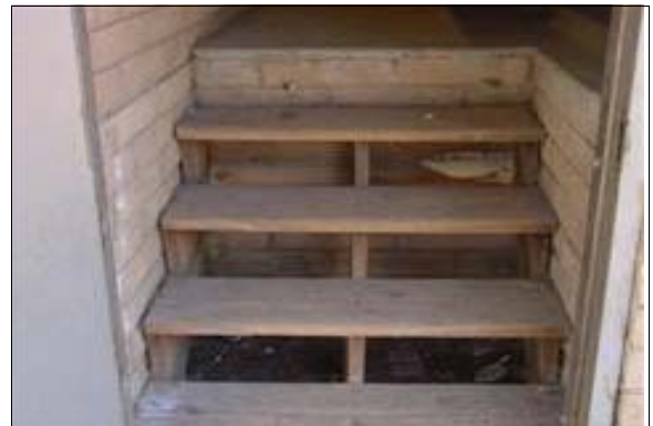
Exterior Stairs to Press Box 1
