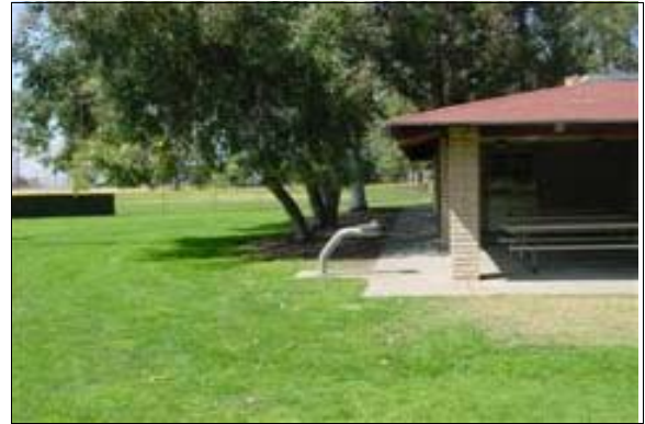
Path of Travel to the Maintenance Building
