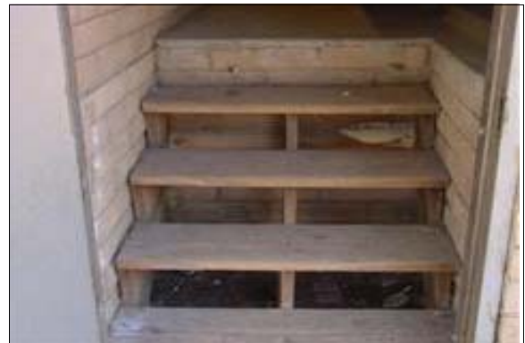
Exterior Stairs to Press Box 1
