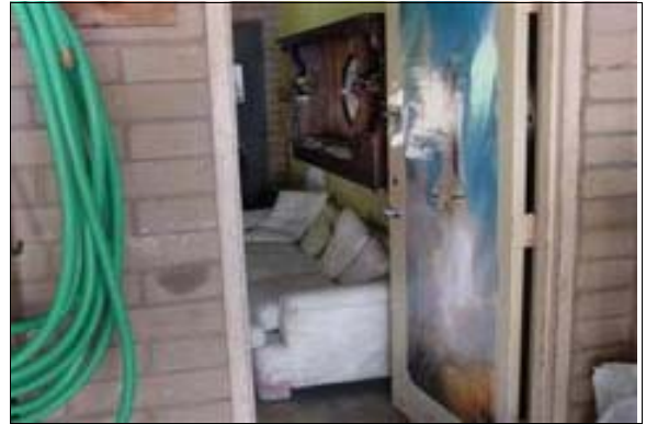
Exterior Door to the Maintenance Office
