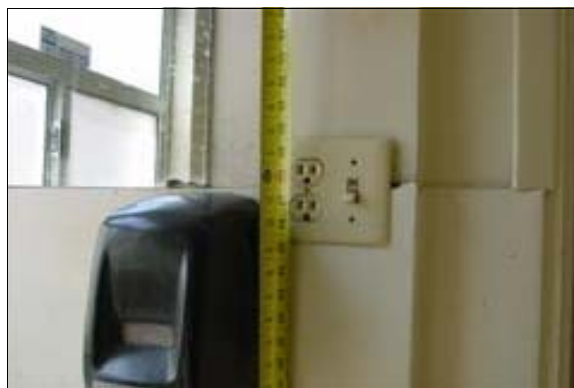
Unisex Restroom at the Maintenance Building
