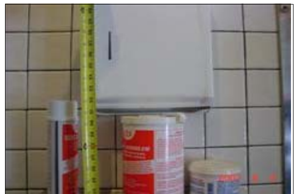
Unisex Restroom in the Maintenance Building
