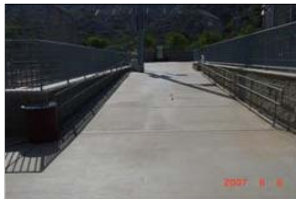
Exterior Ramp Between the Sports Fields
