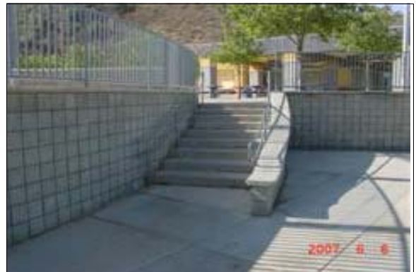
Exterior Stairs to the Outdoor Dining Area
