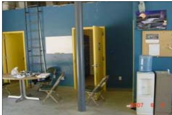
Unisex Restroom in the Maintenance Building
