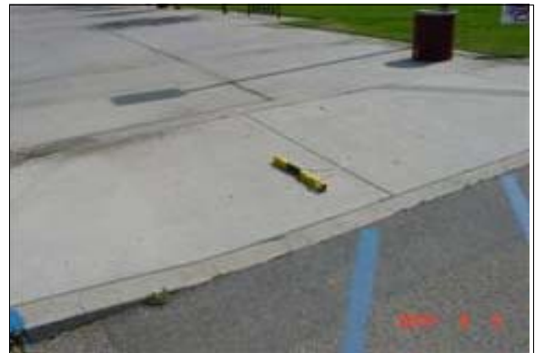
Curb Ramp at the Accessible Parking Spaces Outside of the Office (Right)
