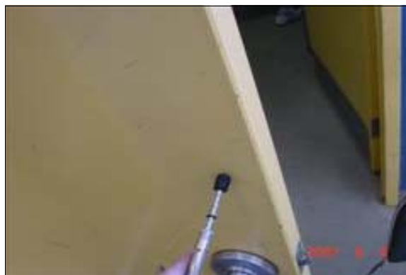
Unisex Restroom in the Maintenance Building
