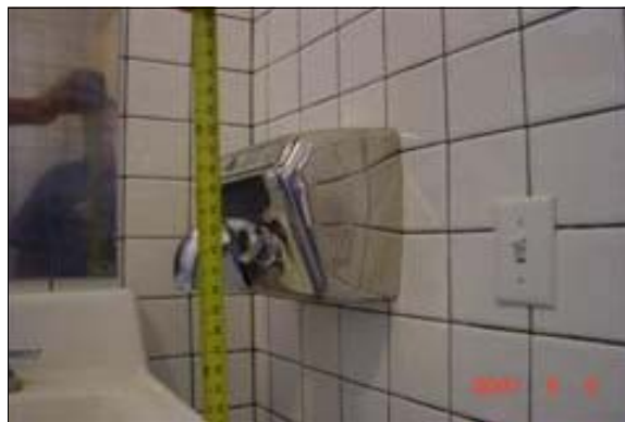
Unisex Restroom in the Maintenance Building
