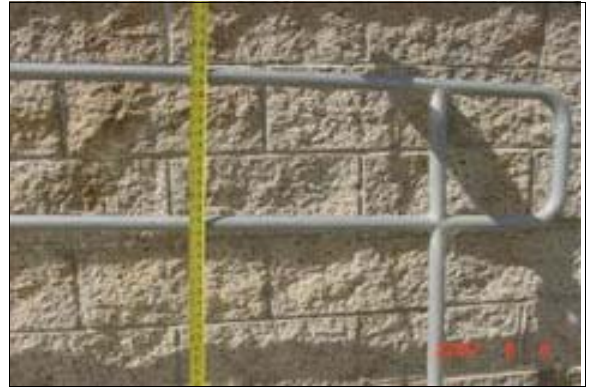
Exterior Ramp Between the Sports Fields
