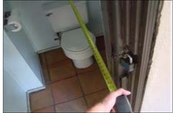
Unisex Restroom at the Rear of the Museum
