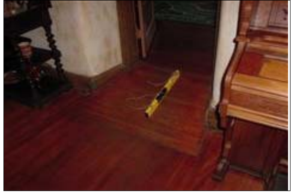
Interior Door to the Dining Area in the Museum
