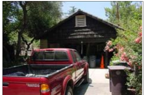
Path of Travel to the Maintenance Garage
