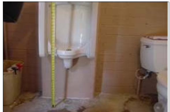
Unisex Restroom at the Maintenance Building
