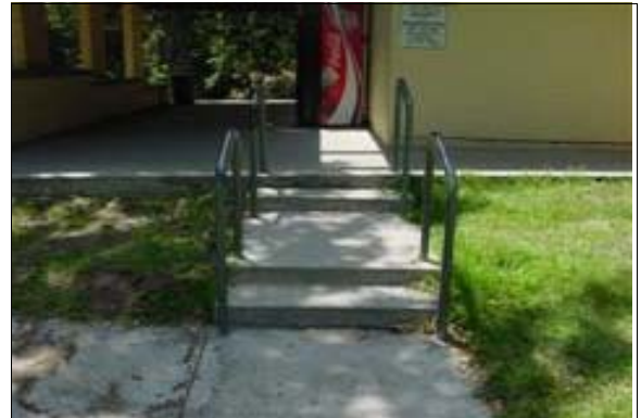
Exterior Stairs to the North Restrooms
