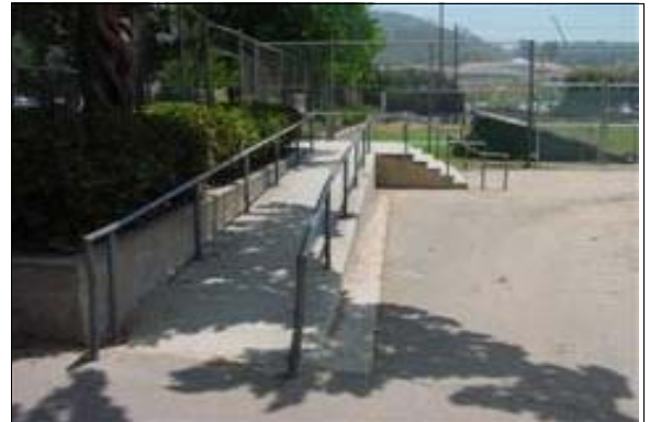
Exterior Ramp to Stengel Field
