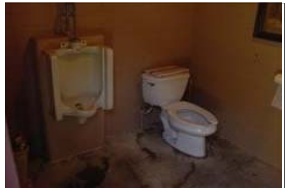
Unisex Restroom at the Maintenance Building
