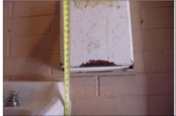
Unisex Restroom at the Maintenance Building
