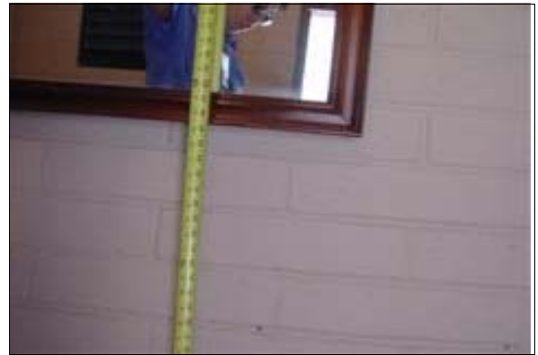
Unisex Restroom at the Maintenance Building
