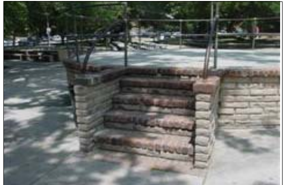
Exterior Stairs to the Outdoor Stage
