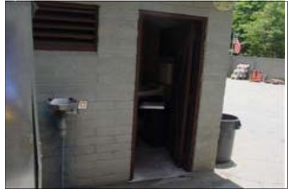
Unisex Restroom at the Maintenance Building
