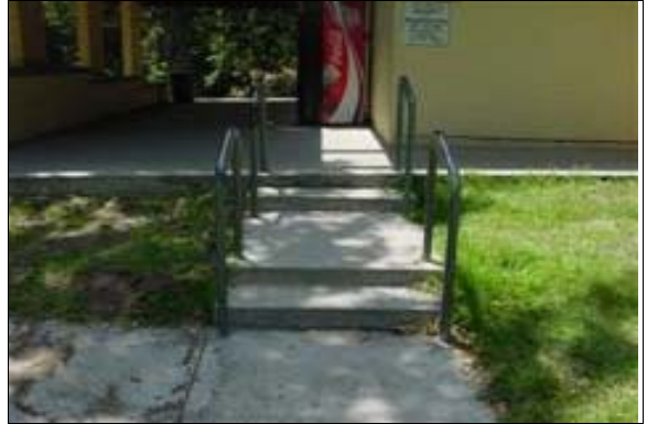
Exterior Stairs to the North Restrooms
