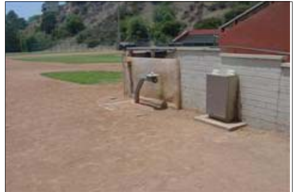
Drinking Fountain at Stengel Field
