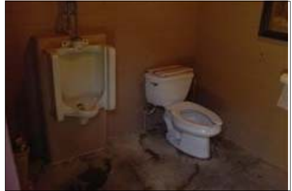
Unisex Restroom at the Maintenance Building
