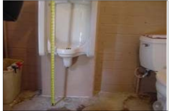
Unisex Restroom at the Maintenance Building
