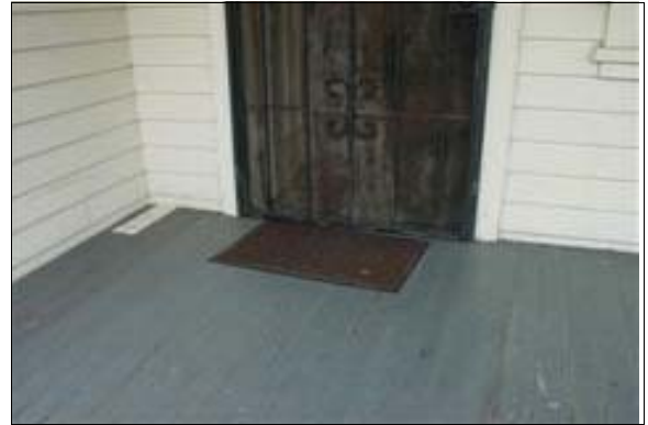
Path of Travel to the Main Entrance
