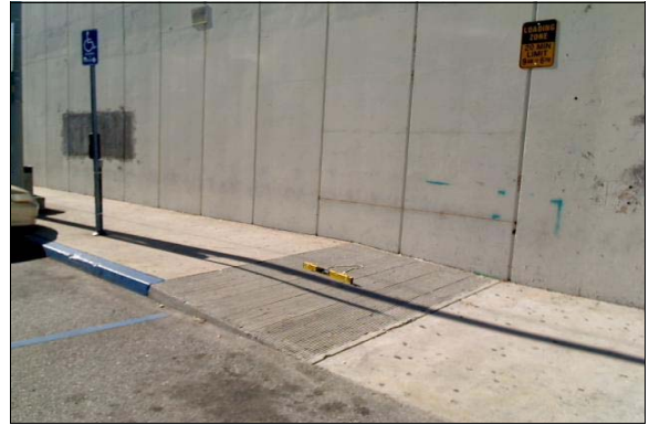
Curb Ramp in front of the Accessible Parking Space
