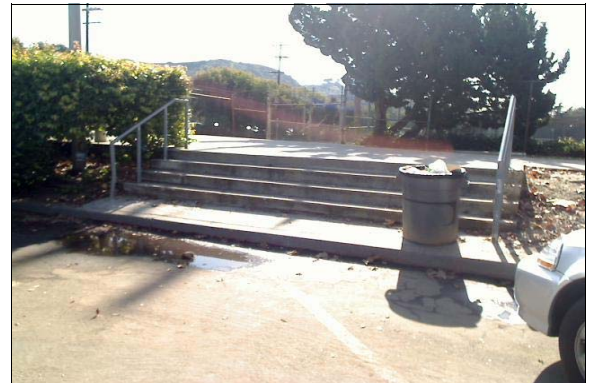
Exterior Stairs to the Public Right of Way
