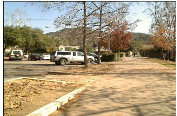
Curb Ramp at the Accessible Parking Access Aisle
